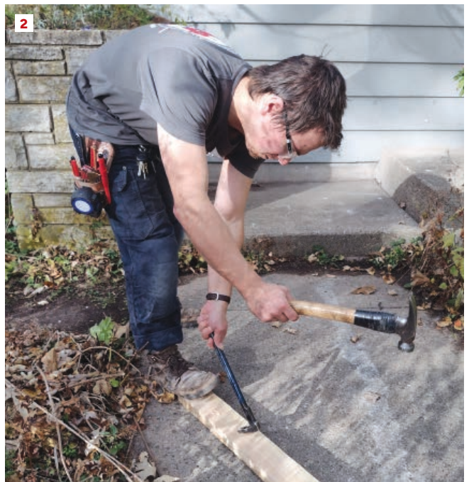
The “V” of the nail puller grabs the nail’s shank, not its brittle head (1, 2).
