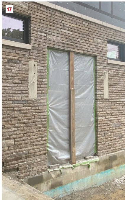
For the gas lanterns, the crew used a combination of pressure treated (PT) lumber (15) and TruExterior 2x10 (16). Thicker PT was required for the mounting blocks that finished flush to the stone (17) than for the blocks that finished flush to the Parklex siding (18).
