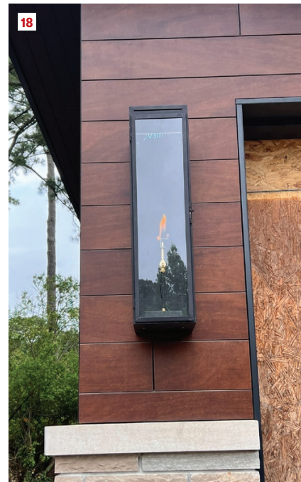
For the gas lanterns, the crew used a combination of pressure treated (PT) lumber (15) and TruExterior 2x10 (16). Thicker PT was required for the mounting blocks that finished flush to the stone (17) than for the blocks that finished flush to the Parklex siding (18).
