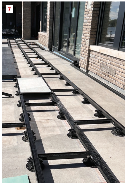
To create a clean joint between tile pavers and stone cladding, the author had concrete block set at the tile elevation as a temporary filler to allow the pavers to slide in beneath the stonework.
