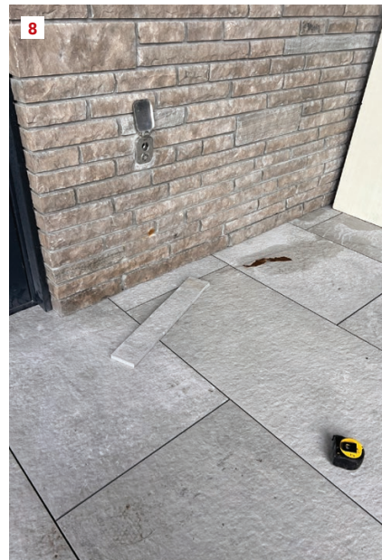
To create a clean joint between tile pavers and stone cladding, the author had concrete block set at the tile elevation as a temporary filler to allow the pavers to slide in beneath the stonework.
