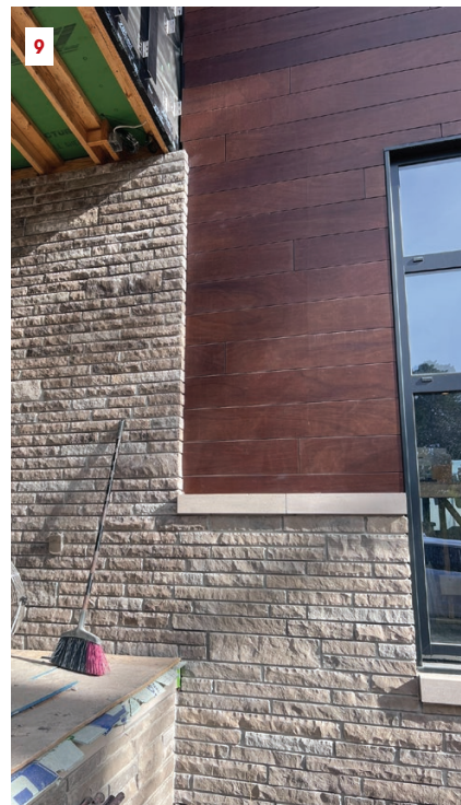
For this vertical transition, the crew had to install the Parklex first, running it long so it would extend behind the stone.
