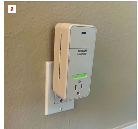
The Broan Overture ventilation control system uses sensors to monitor indoor pollutant levels and ramp up or turn on and off connected ventilation fans to keep pollutant levels at or below threshold levels. The author placed hardwired sensors (1) throughout the living areas and bedrooms. Broan also makes a plug-in sensor (2) that can easily be retrofit in existing outlets.
