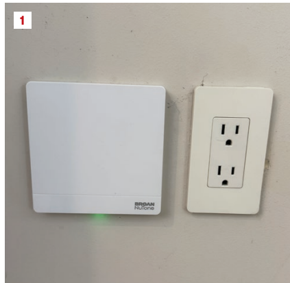
The Broan Overture ventilation control system uses sensors to monitor indoor pollutant levels and ramp up or turn on and off connected ventilation fans to keep pollutant levels at or below threshold levels. The author placed hardwired sensors (1) throughout the living areas and bedrooms. Broan also makes a plug-in sensor (2) that can easily be retrofit in existing outlets.
