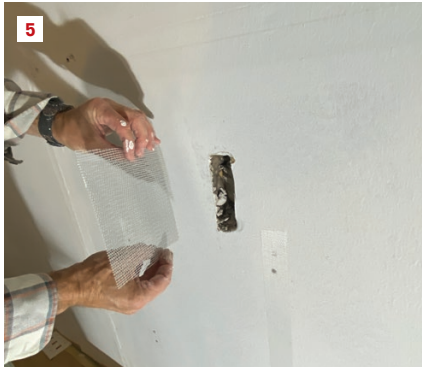
Many screws needed to be reset and some added to secure the drywall again (4). This garage was actively used for storage, which resulted in many dents and holes in the walls. All of them needed to be properly repaired before proceeding (5).
