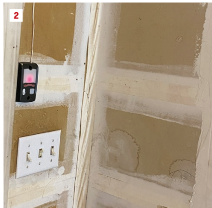
Garage walls yellowed from time and light and marred by water stains, dirt, and failing tape joints are a too common sight for the author (1, 2). To fix the surfaces, he starts by sanding them to clean and prepare the drywall for the next steps (3).
