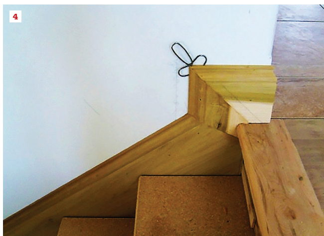
On these stair platforms (1, 2), the baseboards and skirtboards, as well as the profiled cap moldings, are joined with bisected angles. The layout shows how the author resolves a short wall run with a skirt that rises to meet a level baseboard (3, 4).
