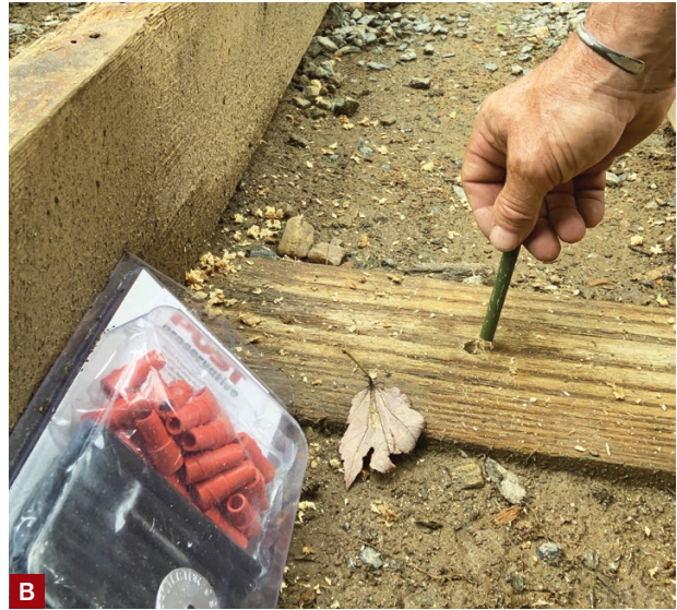
Figure 2. Once the existing framing is exposed, the author reinforces it with structural screws driven through the ledger into the rim joist and blocking as needed (A). To extend the life of the PT framing, the author inserts Post Preservative rods containing a fungicide and wood preservative into holes bored into the wood (B).
