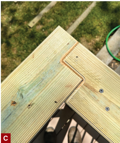
Figure 4. The author temporarily fastens an L-block to a post to hold it in position (A) while he drives structural screws through the post and into the framing (B). On the top rail, the author uses the stepped transition shown here (C) at corners and when joining two top rail sections together mid-span. DekPro aluminum balusters are a low-maintenance alternative to wood balusters and come in both round and square profiles (D).
