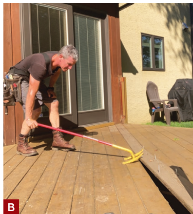
Figure 1. While this home’s existing low-level deck was structurally sound, the western red cedar decking and guard rails needed replacement (A). After removing the rails, the author began prying up the decking from the center, using a NestorBar demolition tool for leverage (B). When the author can’t break off a fastener with a hammer, he cuts it off flush with the framing with an angle grinder (C).
