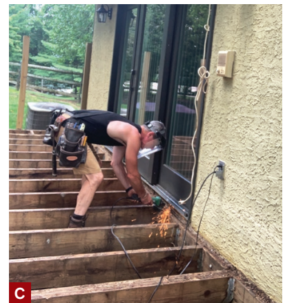
Figure 1. While this home’s existing low-level deck was structurally sound, the western red cedar decking and guard rails needed replacement (A). After removing the rails, the author began prying up the decking from the center, using a NestorBar demolition tool for leverage (B). When the author can’t break off a fastener with a hammer, he cuts it off flush with the framing with an angle grinder (C).
