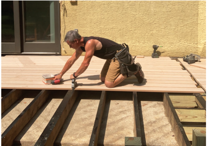
Figure 3. After covering the tops of the joists with self-adhering flashing tape, the author installs the new decking. On this project, he used Modern Mill's Acre decking, a composite material made from upcycled rice hulls and PVC that can be cut like wood and can be stained or painted.
