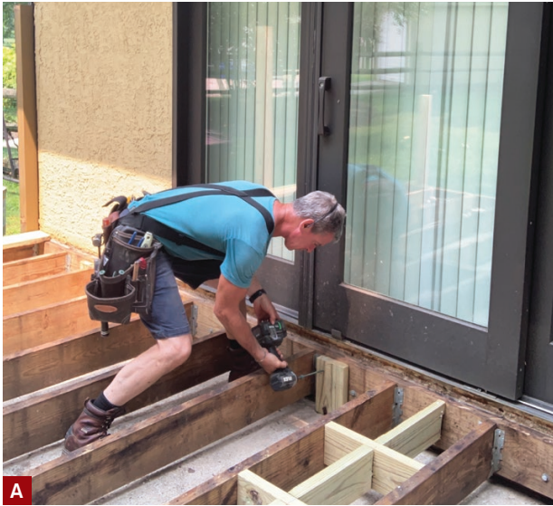
Figure 2. Once the existing framing is exposed, the author reinforces it with structural screws driven through the ledger into the rim joist and blocking as needed (A). To extend the life of the PT framing, the author inserts Post Preservative rods containing a fungicide and wood preservative into holes bored into the wood (B).
