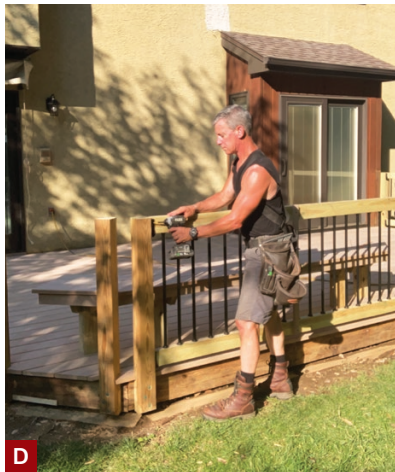
Figure 4. The author temporarily fastens an L-block to a post to hold it in position (A) while he drives structural screws through the post and into the framing (B). On the top rail, the author uses the stepped transition shown here (C) at corners and when joining two top rail sections together mid-span. DekPro aluminum balusters are a low-maintenance alternative to wood balusters and come in both round and square profiles (D).
