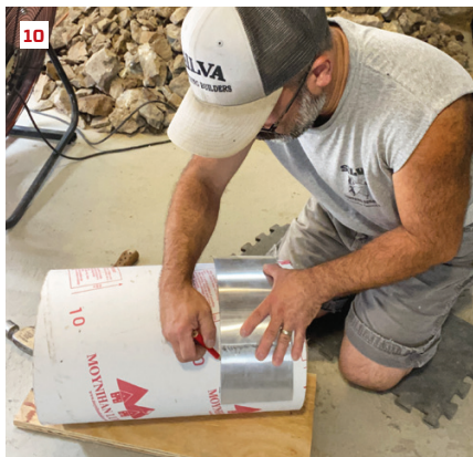
The author drilled holes in the large rocks remaining embedded beneath the slab (7) for 1/2-inch rebar dowels (8) and epoxy adhesive (9) to pin the new footings to the subbase. To form raised piers, he carefully cut 10-inch-diameter tube forms into 6-inch lengths (10) prior to mixing up bags of concrete and filling the holes (11). Only one of the footing holes was rock-free; here, the author reinforced the concrete footing with a rebar grid placed about a third of the depth of the hole (12).
