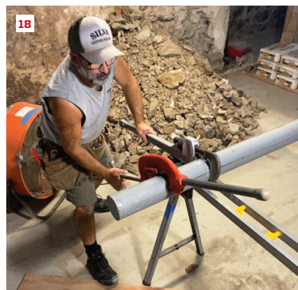
The author inserts a cardboard tube footing form into the wet concrete (13), centering it with a weighted string fastened to the beam above (14). After filling the form with concrete, inserting rebar, and leveling the form (15), he screeded and troweled the top of the pier smooth (16). A pair of overlapping 2x4s (17) were used to get an accurate length for cutting the new column to fit (18).
