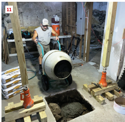
The author drilled holes in the large rocks remaining embedded beneath the slab (7) for 1/2-inch rebar dowels (8) and epoxy adhesive (9) to pin the new footings to the subbase. To form raised piers, he carefully cut 10-inch-diameter tube forms into 6-inch lengths (10) prior to mixing up bags of concrete and filling the holes (11). Only one of the footing holes was rock-free; here, the author reinforced the concrete footing with a rebar grid placed about a third of the depth of the hole (12).
