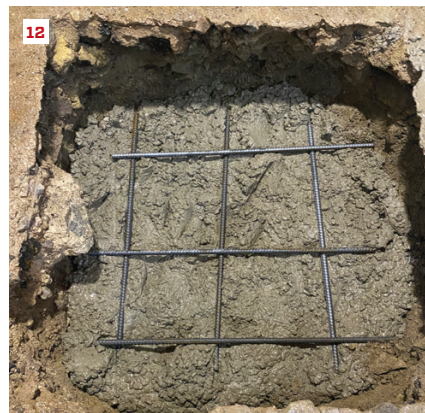
The author drilled holes in the large rocks remaining embedded beneath the slab (7) for 1/2-inch rebar dowels (8) and epoxy adhesive (9) to pin the new footings to the subbase. To form raised piers, he carefully cut 10-inch-diameter tube forms into 6-inch lengths (10) prior to mixing up bags of concrete and filling the holes (11). Only one of the footing holes was rock-free; here, the author reinforced the concrete footing with a rebar grid placed about a third of the depth of the hole (12).
