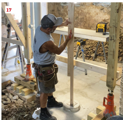
The author inserts a cardboard tube footing form into the wet concrete (13), centering it with a weighted string fastened to the beam above (14). After filling the form with concrete, inserting rebar, and leveling the form (15), he screeded and troweled the top of the pier smooth (16). A pair of overlapping 2x4s (17) were used to get an accurate length for cutting the new column to fit (18).
