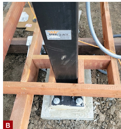
Figure 5. The deck is framed around the steel columns (A, B). The tube-steel rafters are bolted to welded brackets on both sides of the beam (C). Shipping blankets on the beams and the scaffolding protect the steel's powder coating from being scratched during installation.
