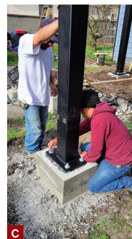
Figure 2. Before the columns are set, concrete is removed from anchor bolt threads and the bottom nuts are screwed on (A). Wiring for lighting is fed through the middle tube-steel post (B). The last of the three factory-welded steel base plates is temporarily set—the upper nuts loosely tightened (C).
