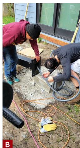
Figure 2. Before the columns are set, concrete is removed from anchor bolt threads and the bottom nuts are screwed on (A). Wiring for lighting is fed through the middle tube-steel post (B). The last of the three factory-welded steel base plates is temporarily set—the upper nuts loosely tightened (C).
