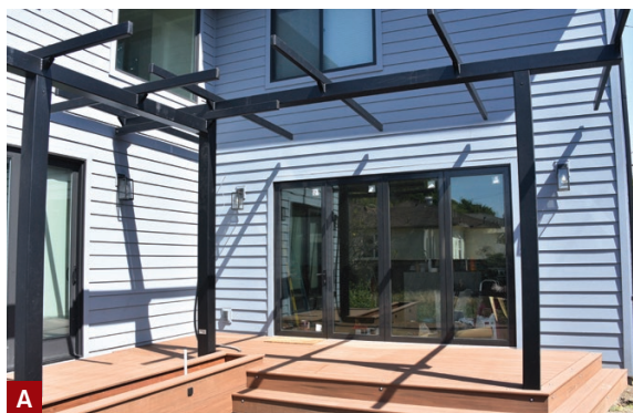
Figure 6. The finished pergola frame (A, B). The homeowner will install canvas-style shading, which will keep afternoon sun from pouring into his kitchen.
