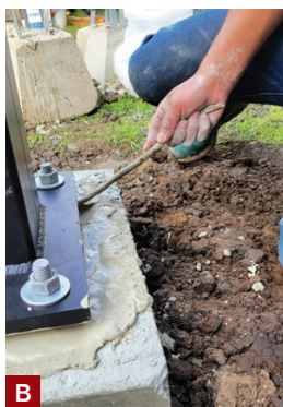
Figure 4. The base plates are set in their final position (A). High-strength grout is packed firmly in place about 1 inch thick to fill any voids (B), then tooled at an angle (C).
