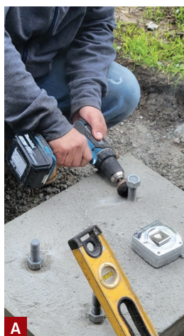
Figure 2. Before the columns are set, concrete is removed from anchor bolt threads and the bottom nuts are screwed on (A). Wiring for lighting is fed through the middle tube-steel post (B). The last of the three factory-welded steel base plates is temporarily set—the upper nuts loosely tightened (C).
