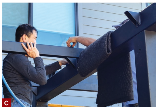
Figure 5. The deck is framed around the steel columns (A, B). The tube-steel rafters are bolted to welded brackets on both sides of the beam (C). Shipping blankets on the beams and the scaffolding protect the steel's powder coating from being scratched during installation.
