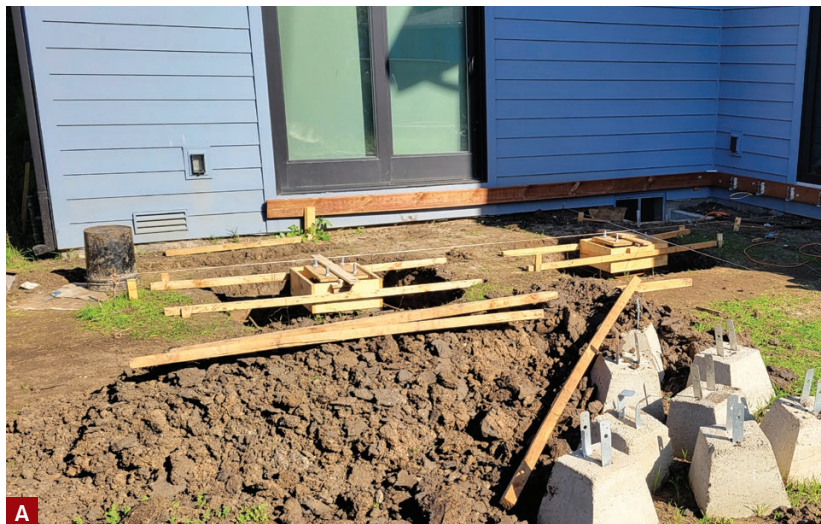
Figure 1. In front of the southwest-facing kitchen, the pergola footings are laid out in a L-shape pattern (A). A raised center section of the footing is formed with 2-by stock nailed to wood supports spanned over the excavated holes. A plywood template precisely holds four anchor bolts in position during the pour (B). Pea-gravel concrete (3,000 psi) is pumped into place (C).
