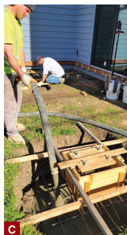
Figure 1. In front of the southwest-facing kitchen, the pergola footings are laid out in a L-shape pattern (A). A raised center section of the footing is formed with 2-by stock nailed to wood supports spanned over the excavated holes. A plywood template precisely holds four anchor bolts in position during the pour (B). Pea-gravel concrete (3,000 psi) is pumped into place (C).
