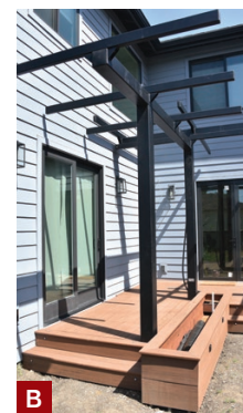
Figure 6. The finished pergola frame (A, B). The homeowner will install canvas-style shading, which will keep afternoon sun from pouring into his kitchen.
