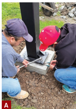
Figure 4. The base plates are set in their final position (A). High-strength grout is packed firmly in place about 1 inch thick to fill any voids (B), then tooled at an angle (C).
