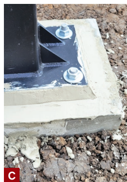
Figure 4. The base plates are set in their final position (A). High-strength grout is packed firmly in place about 1 inch thick to fill any voids (B), then tooled at an angle (C).
