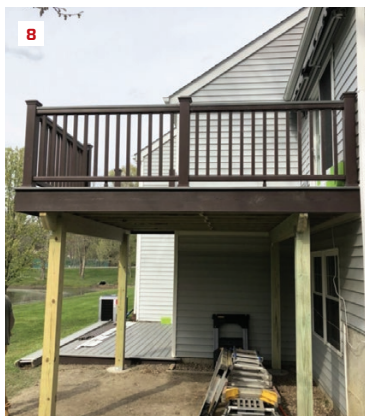
The free-standing deck is supported by a pair of double PT 2x12 drop beams and four 6x6 posts (8). While the condo association approved the new Trex composite decking, the posts and railings needed to be dark brown to match the original deck (9).
