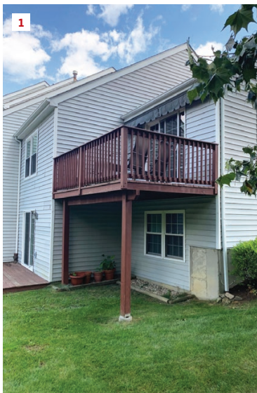
While the existing deck displayed no outward signs of instability (1) , the ledgers had not been properly flashed and the underlying OSB sheathing was revealed to be water damaged upon removal (2) .
