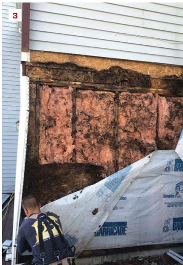
The end-wall sheathing was severely deteriorated (3) , and removing the water-damaged materials revealed that the floor framing had been installed without rim boards; a square hole (top right in photo) was cut into the outboard I-joist to verify floor framing direction (4) .
