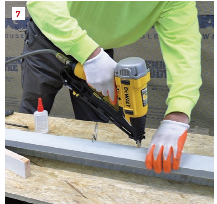
When the author does use corner boards, he preassembles them from \frac{5}{8} -inch TruExterior trim boards. He glues the miter with Dap's RapidFuse adhesive (5, 6), then clamps and nails off the joint (7).
