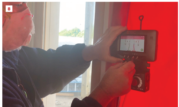
The authors used a new TEC DG-1000 manometer—here compared with an older DG 700 manometer—for the blower door test (7). The DG 1000 is much more intuitive, graphically showing where to connect red and green diagnostic tubing (8).
