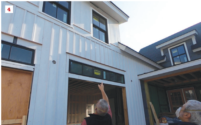
With the building pressurized, fog could be seen escaping from two doghouse dormers at their roof-to-wall junctures (3).
