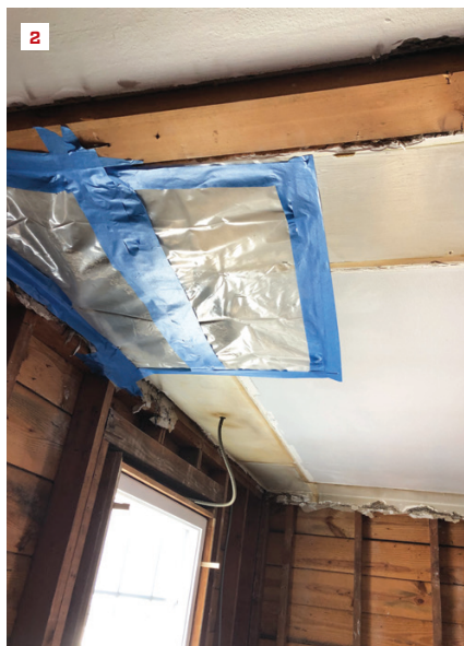
“Before” image of the kitchen in the client’s late-1950s Cape-style home (1). Work stopped when vermiculite was found in the ceiling; the author quickly sealed off the demo hole and around a ceiling light after its discovery (2). A temporary 2-by wall was framed in the middle of an archway to isolate the kitchen and to allow access to the bathroom, bedrooms, and basement (3).
