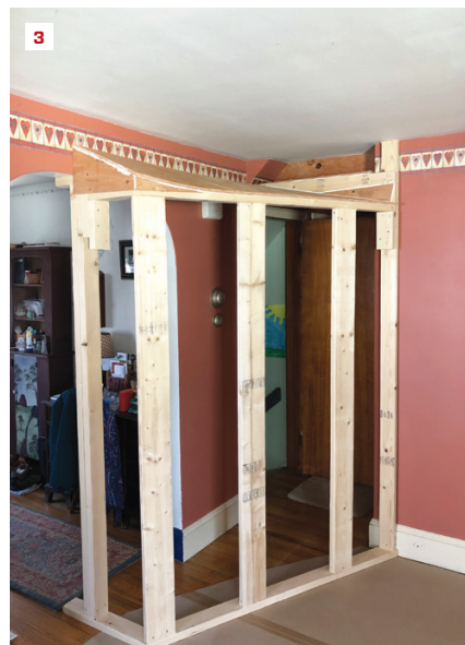
“Before” image of the kitchen in the client’s late-1950s Cape-style home (1). Work stopped when vermiculite was found in the ceiling; the author quickly sealed off the demo hole and around a ceiling light after its discovery (2). A temporary 2-by wall was framed in the middle of an archway to isolate the kitchen and to allow access to the bathroom, bedrooms, and basement (3).
