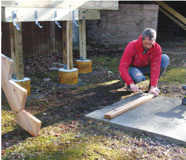
Figure 1. After pouring the concrete for the strip footing and stair landing, the author uses anchor bolts to connect a 2-by PT cleat to the footing (above left). When installing the end stringers, he fastens them to the cleat with structural screws (above right). The middle stringers will be notched to fit over the cleat.
