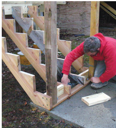
Figure 2. The author screws the guard posts to the stringers (above left), then installs a row of blocking that fits tightly between the stringers (above center). A 1/2-inch-diameter galvanized threaded rod that fits through prebored holes in the posts and stringers ties the assembly together (above right).
