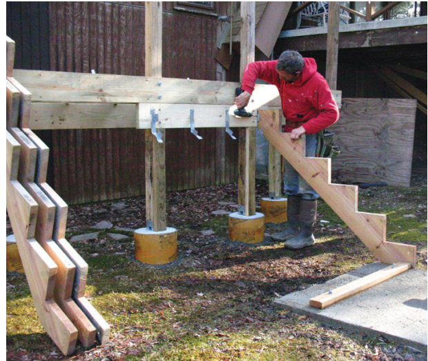
Figure 1. After pouring the concrete for the strip footing and stair landing, the author uses anchor bolts to connect a 2-by PT cleat to the footing (above left). When installing the end stringers, he fastens them to the cleat with structural screws (above right). The middle stringers will be notched to fit over the cleat.
