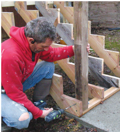
Figure 2. The author screws the guard posts to the stringers (above left), then installs a row of blocking that fits tightly between the stringers (above center). A 1/2-inch-diameter galvanized threaded rod that fits through prebored holes in the posts and stringers ties the assembly together (above right).
