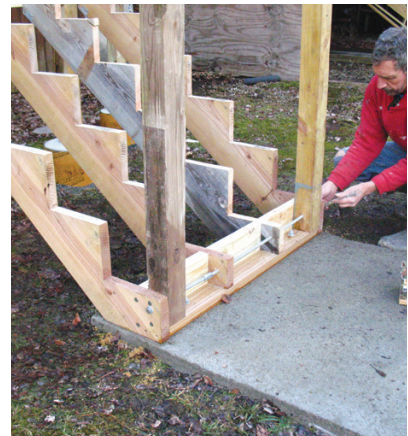
Figure 2. The author screws the guard posts to the stringers (above left), then installs a row of blocking that fits tightly between the stringers (above center). A 1/2-inch-diameter galvanized threaded rod that fits through prebored holes in the posts and stringers ties the assembly together (above right).
