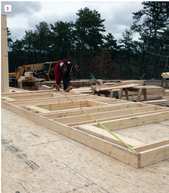
Equal diagonal measurements between the corners ensure that the wall is square (1). The crew then tacks the sheathing to the studs, using a tape measure to follow the layout (2). The sheets are flush with the top plate and split a stud on this home (3).
