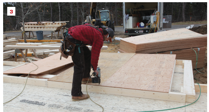
Equal diagonal measurements between the corners ensure that the wall is square (1). The crew then tacks the sheathing to the studs, using a tape measure to follow the layout (2). The sheets are flush with the top plate and split a stud on this home (3).
