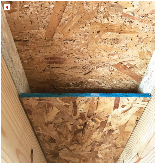
The 1 1/2-inch vent channel terminates in the vented attic of the building (4). Spray foam is applied to the underside of the vent channel (5). If there are imperfections in the spray-foam application, the vent provides backup to clear any moisture.
