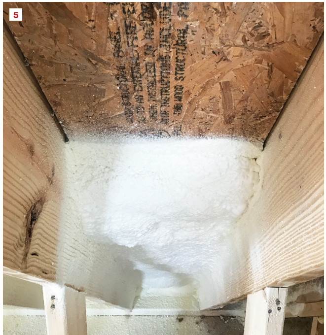
The 1 1/2-inch vent channel terminates in the vented attic of the building (4). Spray foam is applied to the underside of the vent channel (5). If there are imperfections in the spray-foam application, the vent provides backup to clear any moisture.
