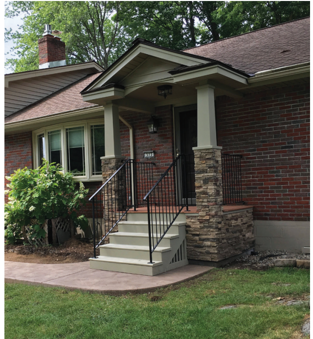
Figure 3. Tapered PVC column wraps dress up the triple 2x6 posts that support the gabled porch roof, which features nicely detailed cornice returns (above left). Along with a new poured concrete walkway and slip-resistant stair treads, the covered porch creates a safe and welcoming entry to the home (above right).
