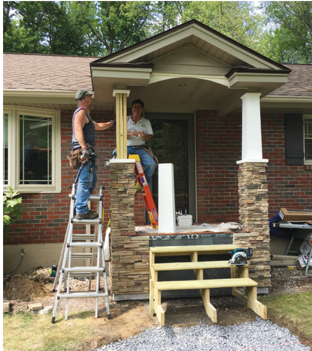
Figure 3. Tapered PVC column wraps dress up the triple 2x6 posts that support the gabled porch roof, which features nicely detailed cornice returns (above left). Along with a new poured concrete walkway and slip-resistant stair treads, the covered porch creates a safe and welcoming entry to the home (above right).
