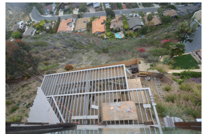
The deck (left) is anchored to the hillside by custom-fabricated galvanized steel support posts, which bear on 12-foot-deep piers (top). Keeping tools and materials from sliding down the hill into neighboring houses was a high priority (bottom).
