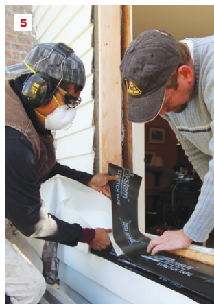
Complex interior trim (1) necessitated removing the 150-year-old windows from the exterior (2). New 2-by stock padded out the R.O. (3), while the sill “pan” was made from flashing tape products (4, 5). A bead of sealant acts as a back dam (6).
