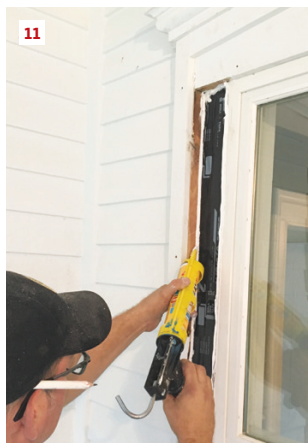
The window unit is lifted in place (7), its frame partially disassembled for access to fastening points (8). A shim screw is used to micro-adjust the jamb (9). The window is reassembled (10), then sealant and trim are applied (11, 12).
