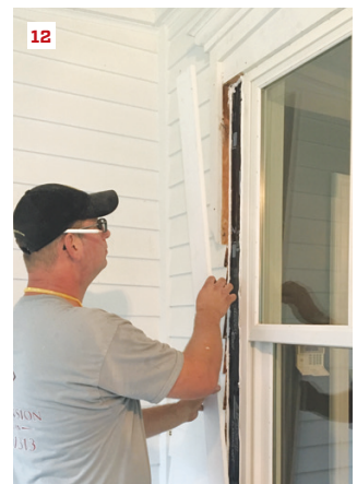
The window unit is lifted in place (7), its frame partially disassembled for access to fastening points (8). A shim screw is used to micro-adjust the jamb (9). The window is reassembled (10), then sealant and trim are applied (11, 12).
