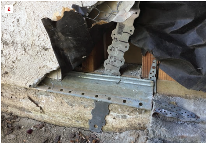
Working from the inside, the author probed with a strap tie to reveal the worst leaks in the house at the bottom plates (1) . At one place, where an exterior door was being replaced, the complete path of the air leaking into the wall cavity is revealed (2) . During an early blower-door test, the air flowing through this outlet and from the crack at the base of the wall gushed air (3) .
