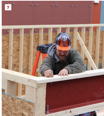
Controlling the heavy steel beam with a tag line, the crew gently lowers it into place across the garage door opening (4). A carpenter marks the 2x6 plate for a bolt hole (5); the plate is then drilled (6) and bolted down to the steel beam (7). A crew member attaches a lifting strap to a PSL beam in preparation for lifting the beam onto the walls (8).
