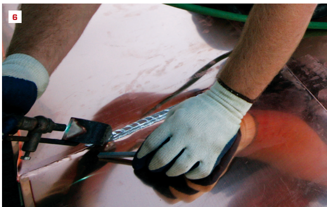
A weighted dead-blow hammer is used to flatten the seams (4). Uphill pans overlap the edges of lower pans (5). Only install as much copper as you can solder in a day (6). The acid from the flux must be neutralized, or it could cause the copper to prematurely (and unevenly) patina (7).
