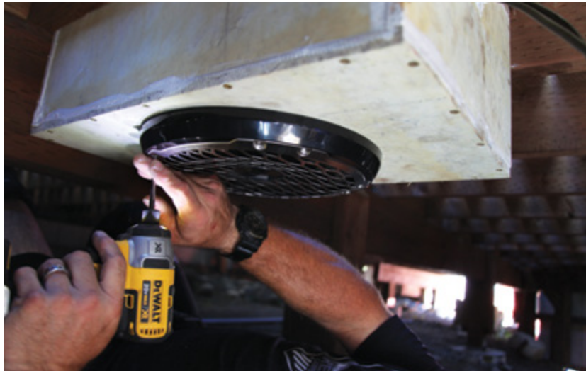
Figure 4. The subwoofer is mounted in a waterproof enclosure underneath the deck. The author built the enclosure with Nylosheet, a waterproof material made of fiberglass and recycled carpet (nyloboard.com).
