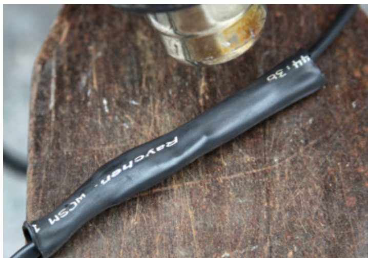
Figure 5. To make weatherproof electrical connections, the author joins marine-quality cable with heat-shrink butt connectors (top left). After making the connection (top right), he then protects the joint with another length of heat-shrink tubing (above).
