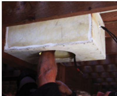
Figure 4. The subwoofer is mounted in a waterproof enclosure underneath the deck. The author built the enclosure with Nylosheet, a waterproof material made of fiberglass and recycled carpet (nyloboard.com).
