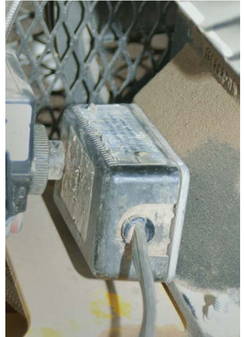
Figure 3. A magnetic oil-pan heater prevents the oil in a compressor from becoming so viscous the machine can't start.
