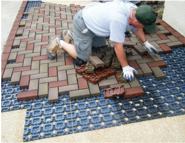
Figure 1. Azek's lightweight pavers are made from old tires and recycled plastic and are installed over a plastic grid system, which locks the pavers in place.
