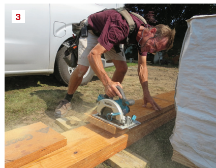
1. The 6 1/2-inch Milwaukee can cut through a 2-by at a 45-degree bevel. 2. Unlike the Makita, the Milwaukee has a built-in rafter hook. 3. The author did some serious framing using the 7 1/4-inch Makita, including trimming LVLs.
