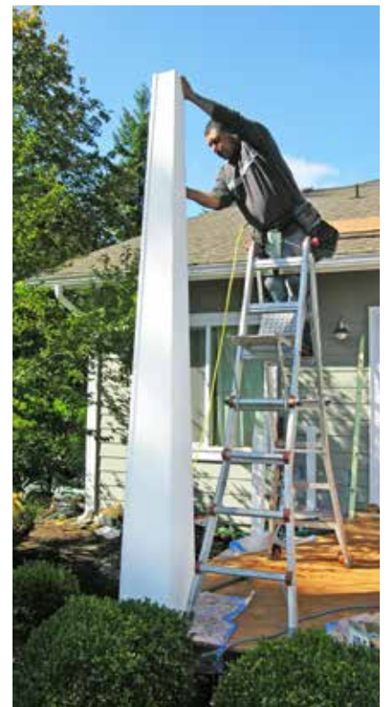
Figure 5. Blocking around the post bases (top) and tapered 2x2s at each corner (above left) provide a frame for the MDO panels that will form the face of the tapered columns. To conceal the rough edges of the panels, 1-by trim is nailed into a bed of caulk at each of the corners (above right).
