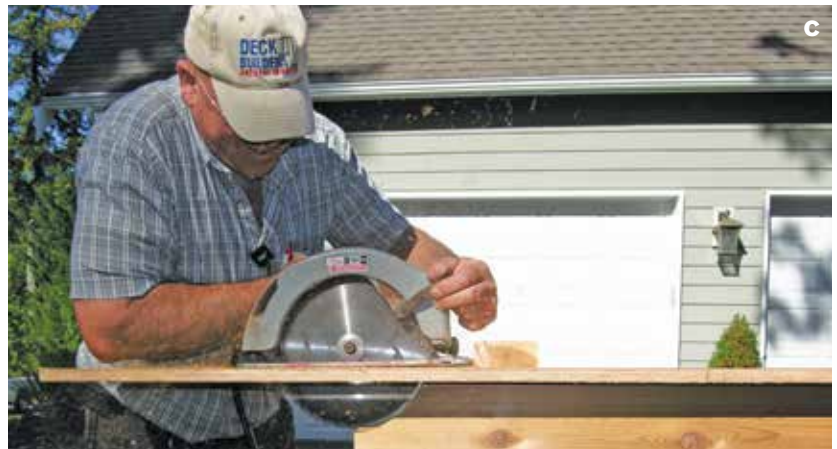
Figure 7. The pergola rafter tails feature a reversed-curve profile. First, the author makes a 45-degree cut at the corner of each rafter to quickly remove excess material (A). Then, guided by a plywood jig (B), the author roughs out the curve with a 10-inch circular saw (C). After smoothing the profile with a sander, the author eases the edges with a round-over bit mounted in a router (D).
