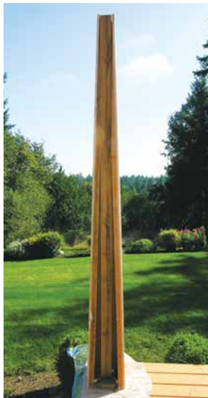
Figure 5. Blocking around the post bases (top) and tapered 2x2s at each corner (above left) provide a frame for the MDO panels that will form the face of the tapered columns. To conceal the rough edges of the panels, 1-by trim is nailed into a bed of caulk at each of the corners (above right).
