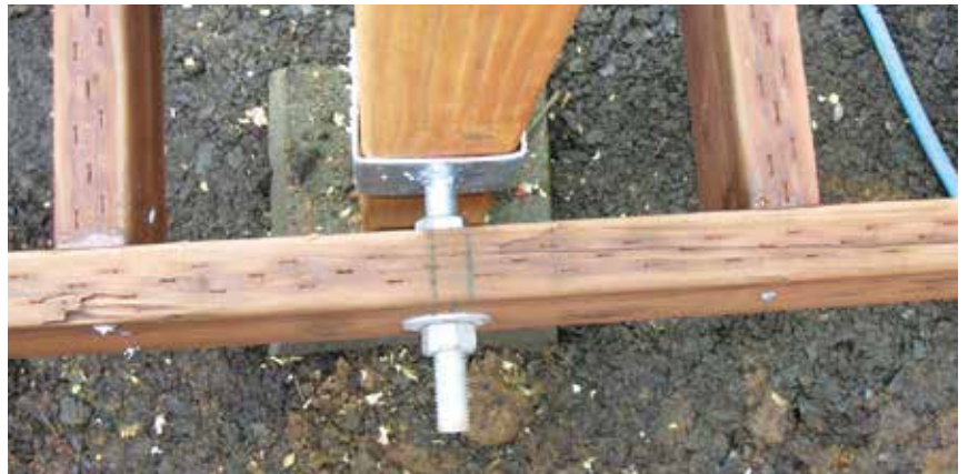
Figure 4. To provide a drying airspace around the posts, the author attaches them to the horizontal framing with post brackets as shown in the two photos above. The bracket's \frac{3}{4} -inch-diameter saddle bolt must be securely fastened with a nut and washer on each side of the joist. Another post bracket (not visible in the photos) attached to a concrete pier keeps each post from contacting the ground.
