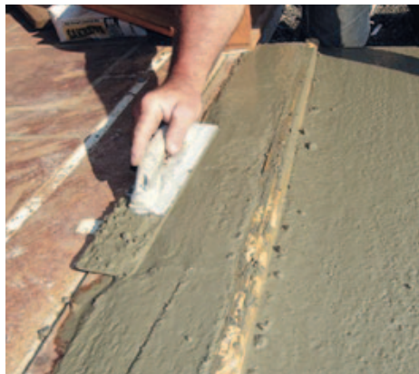
▲ Figure 13. A magnesium float is used where a bull float is too large.
