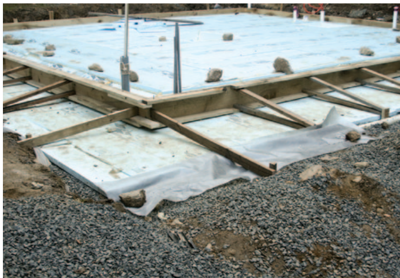
▲ Figure 6. Forms for deeper pours require more bracing.
