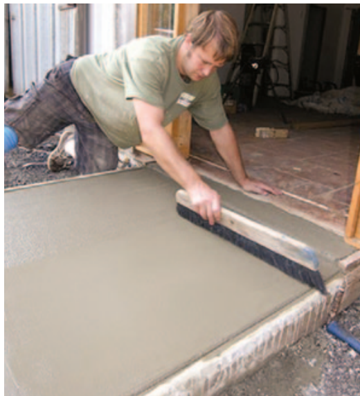
► Figure 19. A slab may be finished with a broom to provide traction.
