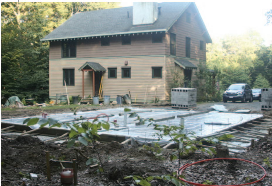
▼ Figure 20. Keep fresh concrete wet for at least 72 hours for at least 72 hours by covering it with plastic or wet burlap, or by continuously running a sprinkler.
