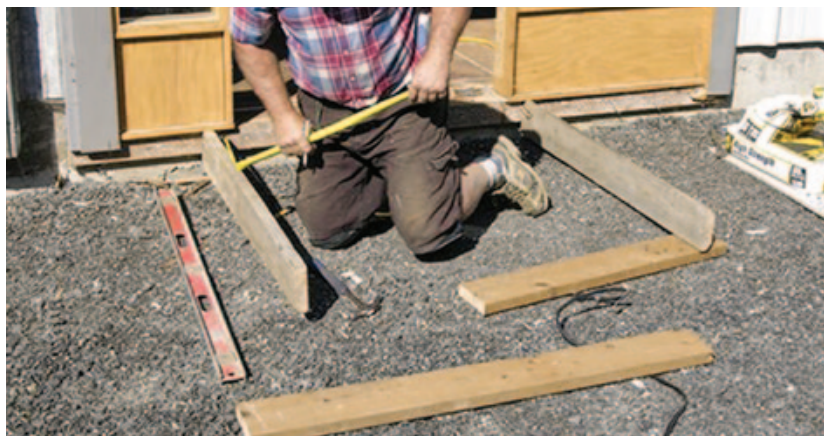
▲ Figure 3. Concrete forms are typically 2x4s nailed together.
