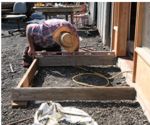
▲ Figure 3. Concrete forms are typically 2x4s nailed together.
