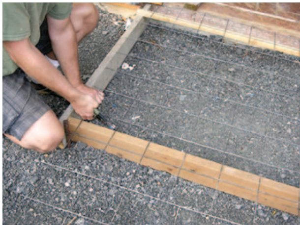
▲ Figure 6. Forms for deeper pours require more bracing.
