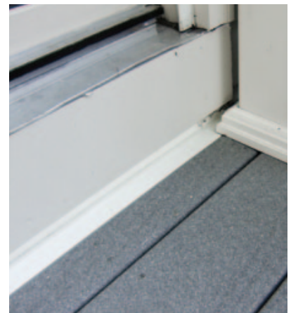
Using a ledger that's one size larger than the joists allows a neat flashing detail (photo, above) and the creation of a drip edge below (illustration, left).
