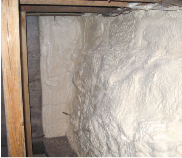
Figure 6. The closed-cell foam on the stone foundation wall at right has been extended a foot or so onto the interior concrete wall at rear to reduce conductive heat loss; the concrete wall was masked before spraying to provide a neat termination. Depending on soils, climate, and other factors, such below-grade applications are sometimes limited to the above-grade portion of the wall — or graduated in thickness, with a thinner layer below grade — to reduce the danger of freezing the footing.
