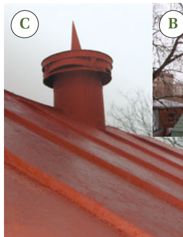
Figure 5. Because it is self-flashing and bonds to a variety of materials, Hydrostop provides seamless coverage between the addition's roof and the brick wall of the main house (A), around the cap of the masonry chimney (B), and between the original metal roof and the vintage vents (C).
