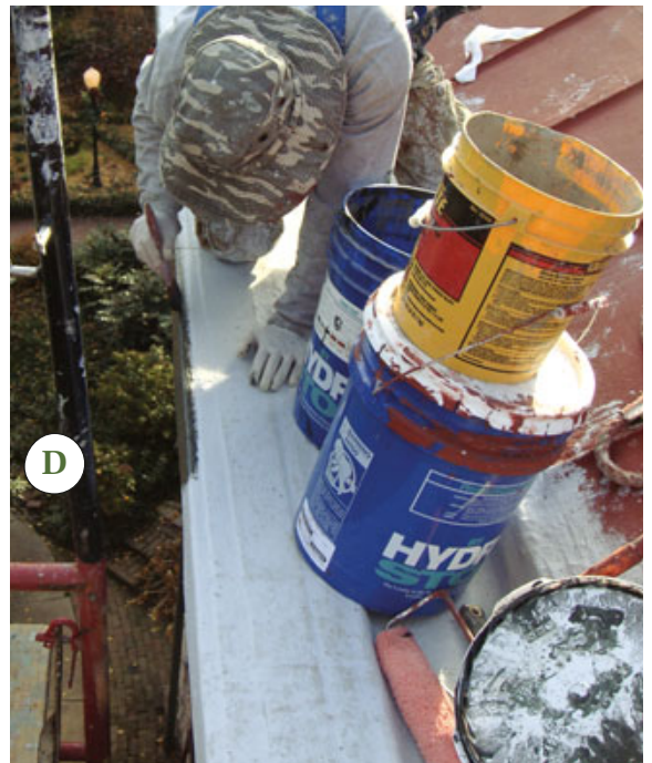
Figure 3. The red finish coat was applied to the seams first (A), then to the field of the roof panels (B). For easy movement over the roof, the installers used ingenious roof-bracket assemblies that hooked over the ridge (C). The existing EPDM-lined gutter was integrated into the new roof surface (D).
