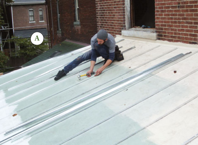
Figure 4. To match the roof of the main house, faux standing seams were added to the plywood roof sheathing on the addition (A and B). Next, the metal and wood surfaces were covered with polyester fabric and a bedding coat (C), followed by two finish coats (D).
