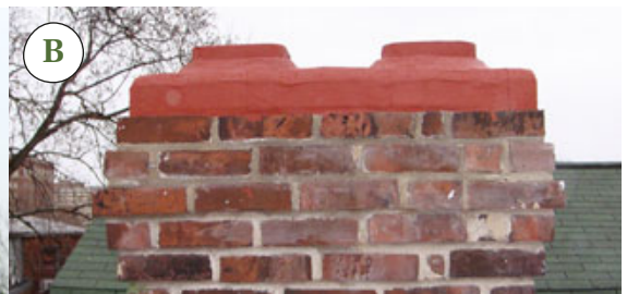
Figure 5. Because it is self-flashing and bonds to a variety of materials, Hydrostop provides seamless coverage between the addition's roof and the brick wall of the main house (A), around the cap of the masonry chimney (B), and between the original metal roof and the vintage vents (C).
