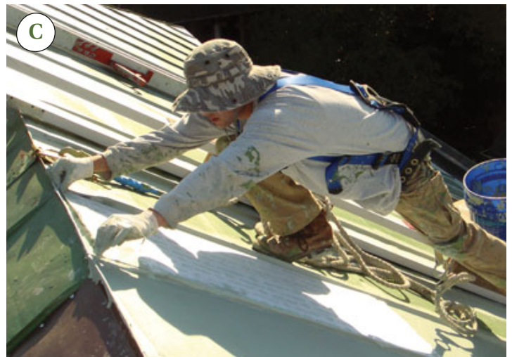
Figure 2. A white bedding coat and polyester fabric followed the green primer (A). The standing seams were treated first, with strips of fabric pressed over the raised profiles into the thick compound (B). The field of the roof was then covered (C). Now the roof was ready for the finish coats (D).
