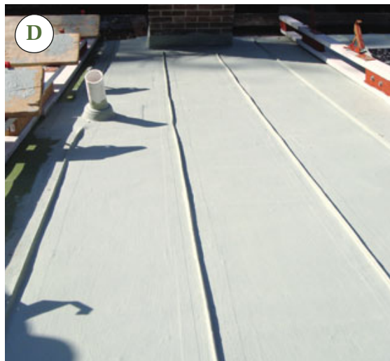
Figure 2. A white bedding coat and polyester fabric followed the green primer (A). The standing seams were treated first, with strips of fabric pressed over the raised profiles into the thick compound (B). The field of the roof was then covered (C). Now the roof was ready for the finish coats (D).
