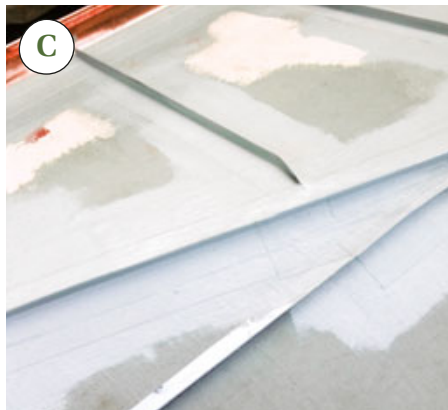
Figure 4. To match the roof of the main house, faux standing seams were added to the plywood roof sheathing on the addition (A and B). Next, the metal and wood surfaces were covered with polyester fabric and a bedding coat (C), followed by two finish coats (D).
