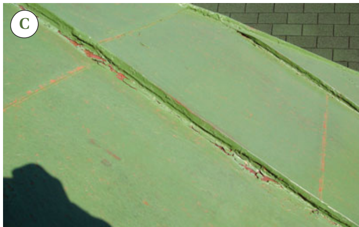
Figure 1. The original painted roof (A) was first pressure-washed (B), then allowed to dry. The contrasting green primer coat that came next (C) revealed areas that needed further attention with a wire brush. Painted sheet aluminum was used to patch holes where vents had been removed (D).
