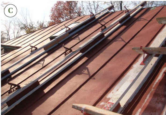
Figure 3. The red finish coat was applied to the seams first (A), then to the field of the roof panels (B). For easy movement over the roof, the installers used ingenious roof-bracket assemblies that hooked over the ridge (C). The existing EPDM-lined gutter was integrated into the new roof surface (D).
