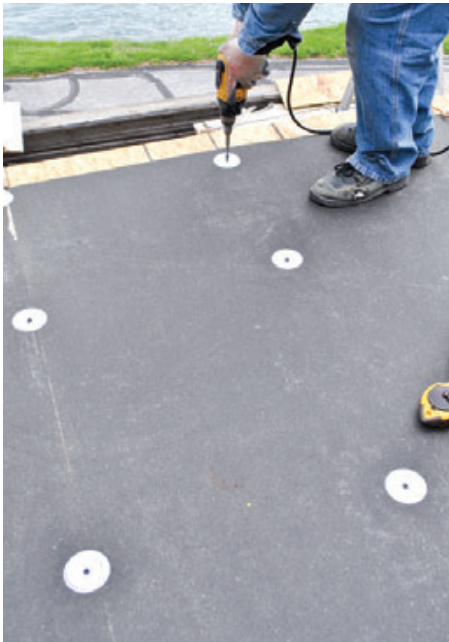
Figure 3. The EPDM installation started with a 1/2-inch-thick fiberboard underlayment engineered to bond with the roofing adhesive. It scores and cuts like cement board and is fastened in place with galvanized screws and washers (above). After sweeping the surface clean, the crew applies latex bonding adhesive, folding the membrane back on itself so it can be glued down a section at a time (right).
