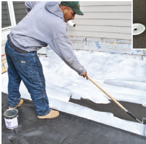
Figure 3. The EPDM installation started with a 1/2-inch-thick fiberboard underlayment engineered to bond with the roofing adhesive. It scores and cuts like cement board and is fastened in place with galvanized screws and washers (above). After sweeping the surface clean, the crew applies latex bonding adhesive, folding the membrane back on itself so it can be glued down a section at a time (right).
