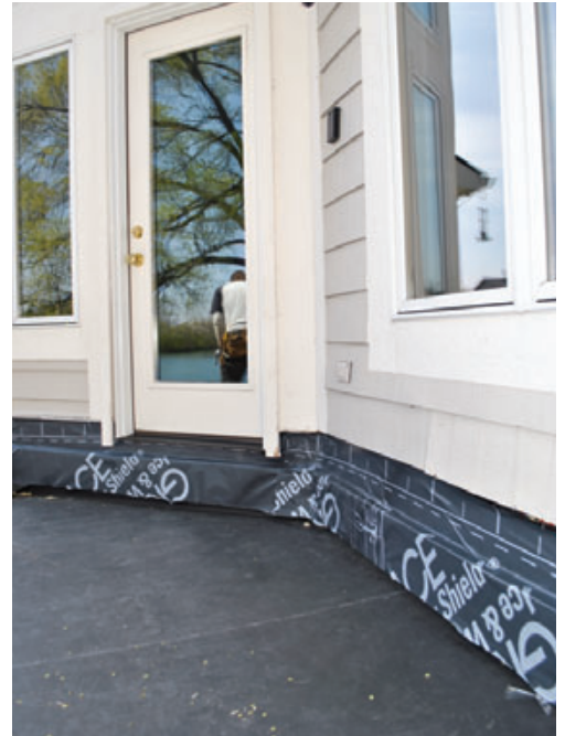
Figure 7. A pressure-treated deck ledger (above left), flashed with Ice & Water Shield (above), supports the inboard end of the new joists. The original decking and railing were reinstalled to complete the roofing job (left).
