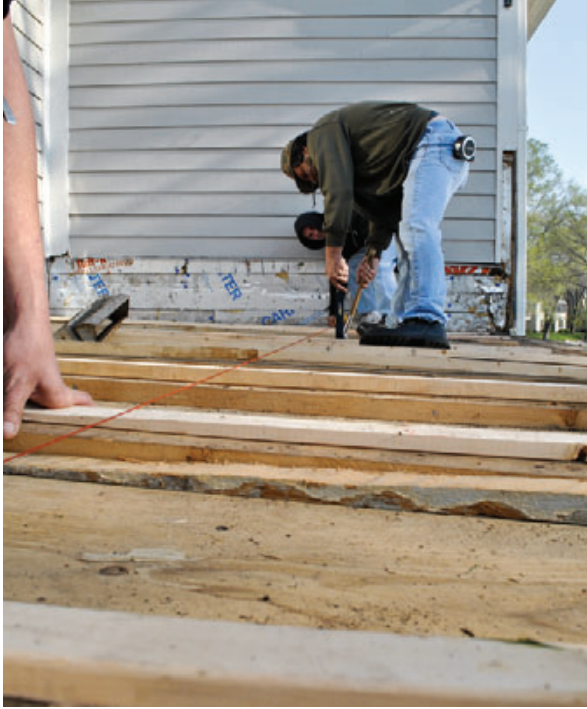
Figure 2. Since the sheathing had to be replaced anyway, the author increased the roof slope by adding tapered 2-by sleepers on top of the joists (left). The new OSB decking slopes 4 inches over 11 feet — an additional 3 inches of rise (above).
