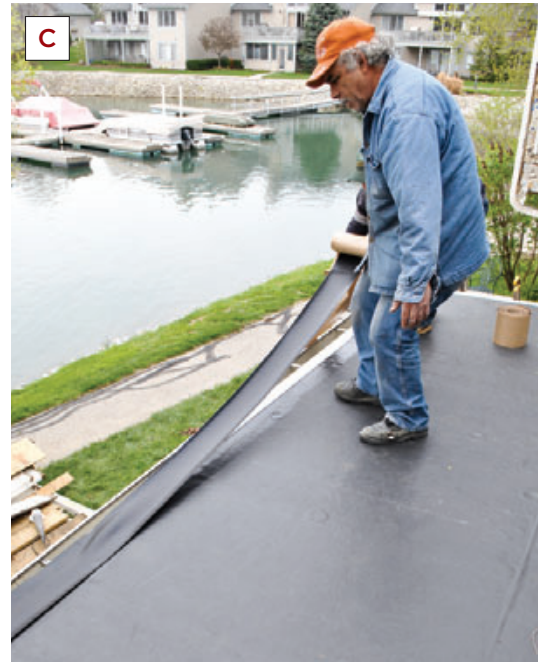
Figure 5. The roofers pull the EPDM tight and tack it in place (A), leaving it long enough to ensure that water flows into — rather than behind — the gutter. The roof edge is protected with a gutter apron. Glue is applied to the apron (B), followed by seam tape (C), which is pressed into place with a rubber roller (D). Although the tape is self-adhering, the author uses glue as an extra precaution.
