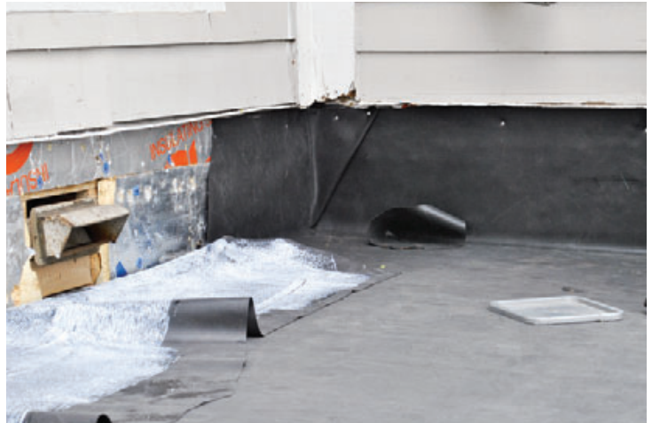
Figure 4. As the cement sets, a worker uses a broom to press out air bubbles and create a strong bond (above left). The membrane is left long, then folded up the wall and trimmed to its final length. To minimize cuts, the corners are folded over (above). After the entire sheet is adhered, brooming continues until all the bubbles are worked out at the upper edge (left).
