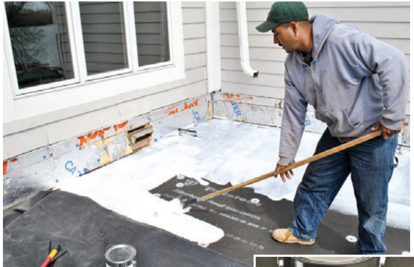
Figure 2. Since the sheathing had to be replaced anyway, the author increased the roof slope by adding tapered 2-by sleepers on top of the joists (left). The new OSB decking slopes 4 inches over 11 feet — an additional 3 inches of rise (above).
