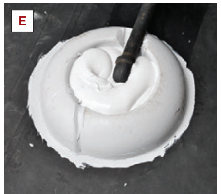
Figure 6. The author seals pipe penetrations with PVC donuts. First the donut is cut in half to fit around the pipe (A), then it's glued to the roof with a pourable sealant (B, C), which is also used to fill the center (D). The cured sealant (E) stays flexible over time so it can adapt to movement in the roof without losing its seal.
