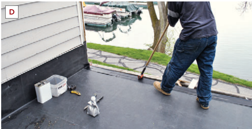
Figure 5. The roofers pull the EPDM tight and tack it in place (A), leaving it long enough to ensure that water flows into — rather than behind — the gutter. The roof edge is protected with a gutter apron. Glue is applied to the apron (B), followed by seam tape (C), which is pressed into place with a rubber roller (D). Although the tape is self-adhering, the author uses glue as an extra precaution.
