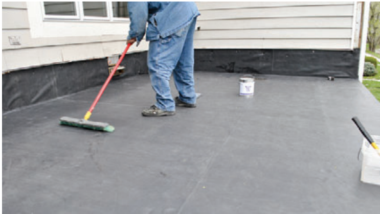
Figure 4. As the cement sets, a worker uses a broom to press out air bubbles and create a strong bond (above left). The membrane is left long, then folded up the wall and trimmed to its final length. To minimize cuts, the corners are folded over (above). After the entire sheet is adhered, brooming continues until all the bubbles are worked out at the upper edge (left).
