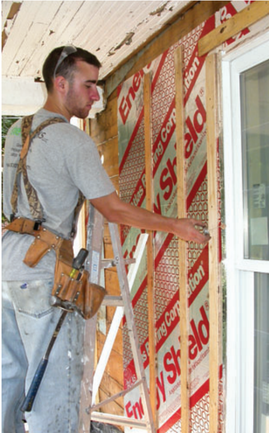
Figure 5. Battens ripped from \frac{3}{8} -inch plywood were fastened through the foam and sheathing into the wall framing to provide solid nailing for the fiber-cement siding and create a drying airspace behind it (left). Strips of \frac{3}{8} -inch-thick Cor-A-Vent installed along the base of the wall between the battens keep out insects (above).
