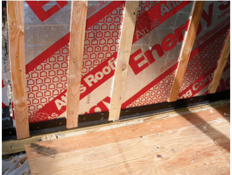
Figure 5. Battens ripped from \frac{3}{8} -inch plywood were fastened through the foam and sheathing into the wall framing to provide solid nailing for the fiber-cement siding and create a drying airspace behind it (left). Strips of \frac{3}{8} -inch-thick Cor-A-Vent installed along the base of the wall between the battens keep out insects (above).
