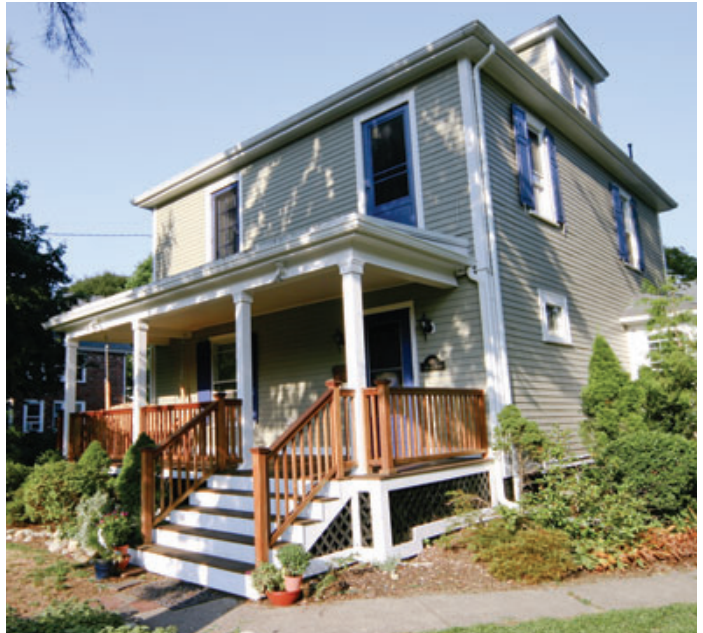
Figure 6. Workers trimmed the corners with one-piece Azek PVC corner boards (left). To reduce maintenance costs, the homeowners opted to replace the weathered cedar shingles with new factory-painted fiber-cement lap siding (above).
