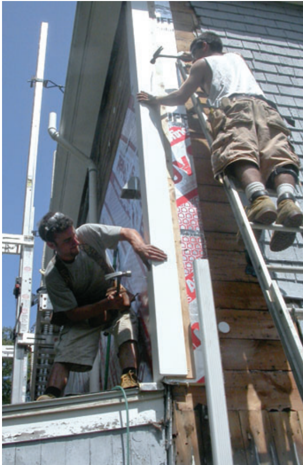
Figure 6. Workers trimmed the corners with one-piece Azek PVC corner boards (left). To reduce maintenance costs, the homeowners opted to replace the weathered cedar shingles with new factory-painted fiber-cement lap siding (above).
