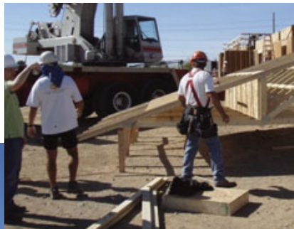
Here’s one way to provide fall protection for leading-edge workers during roof framing: Assemble three or more truss sections on the ground (above) and crane them into position, allowing workers to clip into anchor points pre-installed by the truss manufacturer (left).
