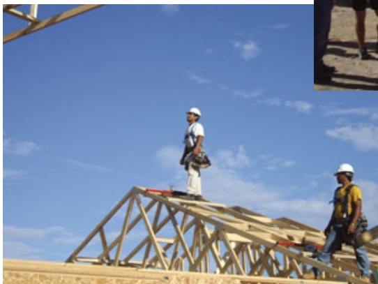
Here’s one way to provide fall protection for leading-edge workers during roof framing: Assemble three or more truss sections on the ground (above) and crane them into position, allowing workers to clip into anchor points pre-installed by the truss manufacturer (left).
