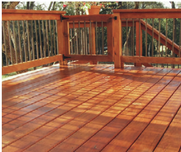
Figure 1. Thermally modified wood takes on a dark color along with its decay-resistant qualities.
