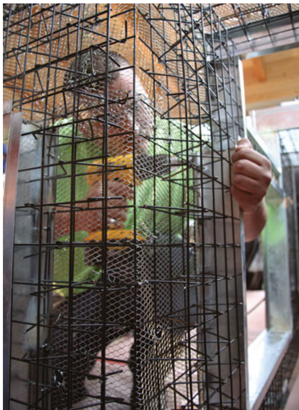
Figure 1. Structural panels made from heavy-gauge galvanized wire form the skeleton of this outdoor kitchen.
