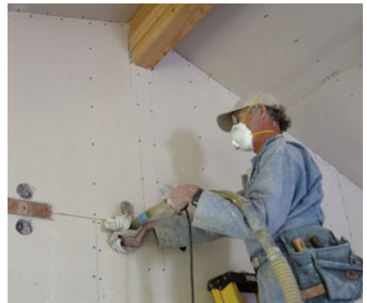
Figure 8. Holes bored in the rafter blocks (left) provided access to the closed framing cavities after the drywall had been hung. The insulation contractor used a long PVC wand — inserted to the end of the cavity and slowly withdrawn as material was blown in — to maintain a consistent density for the full length of the rafter cavities (below left). The remaining cavities were filled from inside the building, after it had been determined that the drywall was dry enough to resist bulging or tearing at the screws (below).
