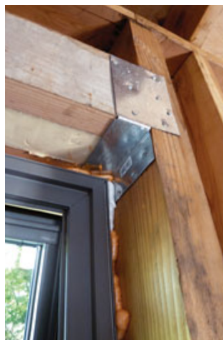
Figure 5. High-solar-gain glazing was used on the south elevation and low-gain glazing on the other sides; U-values range from 0.14 to 0.19. Inside, the units were sealed to the rough opening with spray foam (above left), then surrounded with a thermal break of rigid foam (above right). Later, the drywall was returned into the opening and finished with corner bead.
