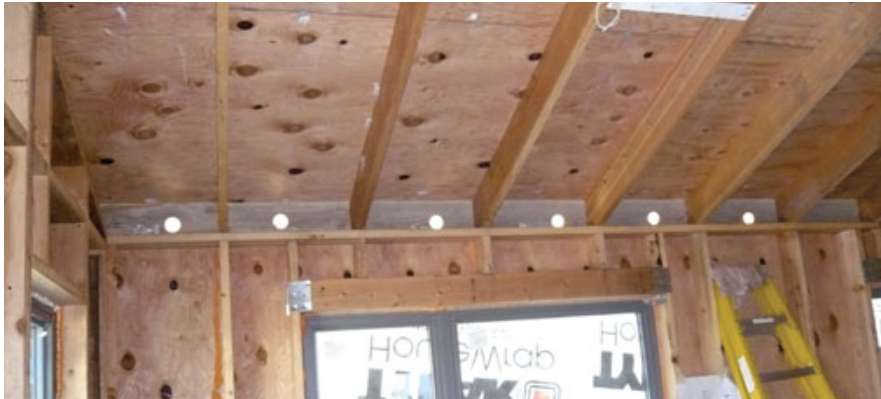
Figure 8. Holes bored in the rafter blocks (left) provided access to the closed framing cavities after the drywall had been hung. The insulation contractor used a long PVC wand — inserted to the end of the cavity and slowly withdrawn as material was blown in — to maintain a consistent density for the full length of the rafter cavities (below left). The remaining cavities were filled from inside the building, after it had been determined that the drywall was dry enough to resist bulging or tearing at the screws (below).
