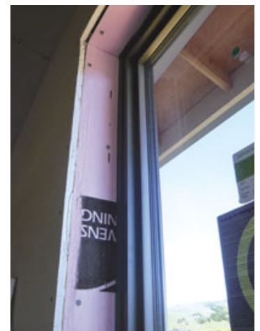
Figure 5. High-solar-gain glazing was used on the south elevation and low-gain glazing on the other sides; U-values range from 0.14 to 0.19. Inside, the units were sealed to the rough opening with spray foam (above left), then surrounded with a thermal break of rigid foam (above right). Later, the drywall was returned into the opening and finished with corner bead.
