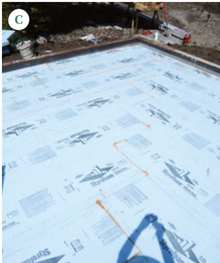
Figure 2. The stone base inside the stem wall was leveled and compacted, then covered with 6-mil poly and 4-inch XPS insulation (A). A layer of 3-inch foam was laid over the first layer (B), with joints staggered and all gaps in both layers filled with spray foam (C). A second layer of poly and steel reinforcing followed (D).
