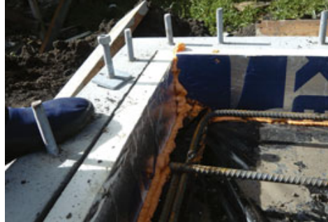
Figure 1. An excavated bed filled with crushed stone served as a base for the stem-wall foundation, which was stepped down at its upper edge so that the exterior foam insulation wrapping the frame would cover the edge of the mudsill, eliminating a potential thermal bypass (far left). A vertical strip of polyiso board around the inside of the stem wall minimizes heat loss at the slab edge (left, top). For air-sealing the frame to the slab, the mudsills were bolted in place in a bed of roofing cement (left, bottom).
