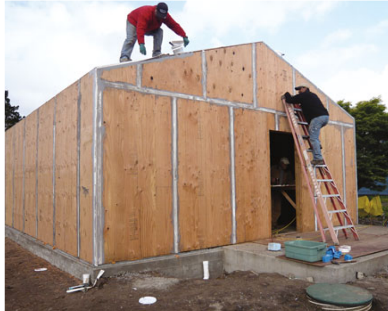
Figure 4. To air-seal the 1/2-inch sheathing to the framing as it was installed, one carpenter laid beads of foam on the framing edges while another followed with a nail gun (left). The plywood seams on both the walls and the roof were further sealed with drywall tape and duct mastic (right).
