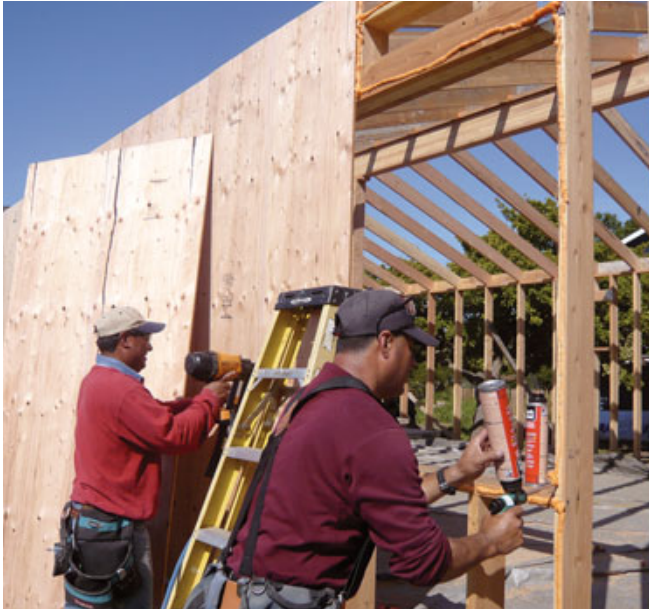
Figure 4. To air-seal the 1/2-inch sheathing to the framing as it was installed, one carpenter laid beads of foam on the framing edges while another followed with a nail gun (left). The plywood seams on both the walls and the roof were further sealed with drywall tape and duct mastic (right).
