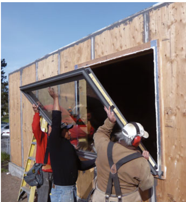
Figure 5. High-solar-gain glazing was used on the south elevation and low-gain glazing on the other sides; U-values range from 0.14 to 0.19. Inside, the units were sealed to the rough opening with spray foam (above left), then surrounded with a thermal break of rigid foam (above right). Later, the drywall was returned into the opening and finished with corner bead.
