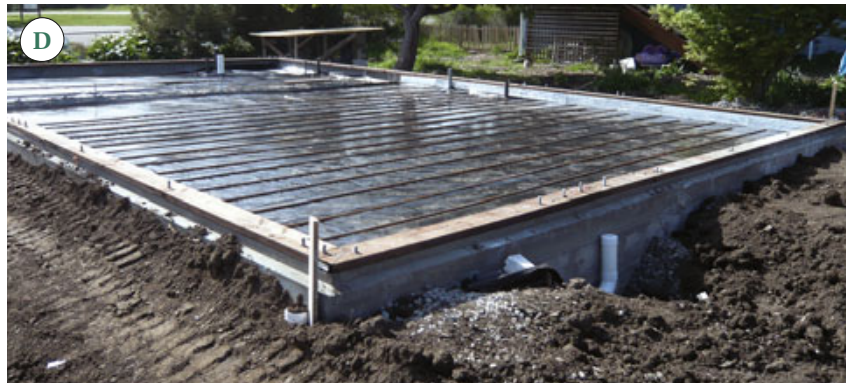
Figure 2. The stone base inside the stem wall was leveled and compacted, then covered with 6-mil poly and 4-inch XPS insulation (A). A layer of 3-inch foam was laid over the first layer (B), with joints staggered and all gaps in both layers filled with spray foam (C). A second layer of poly and steel reinforcing followed (D).
