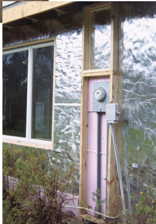
Figure 7. The perimeter of the slab-on-grade addition was insulated with two layers of 1½-inch extruded polystyrene (above left), matching the thickness of the polyiso on the walls (above). Rather than go to the expense of moving the electric meter away from the wall to accommodate the full thickness of the polyiso board, the crew boxed in the area around the meter and filled it with a thinner layer of XPS (left).
