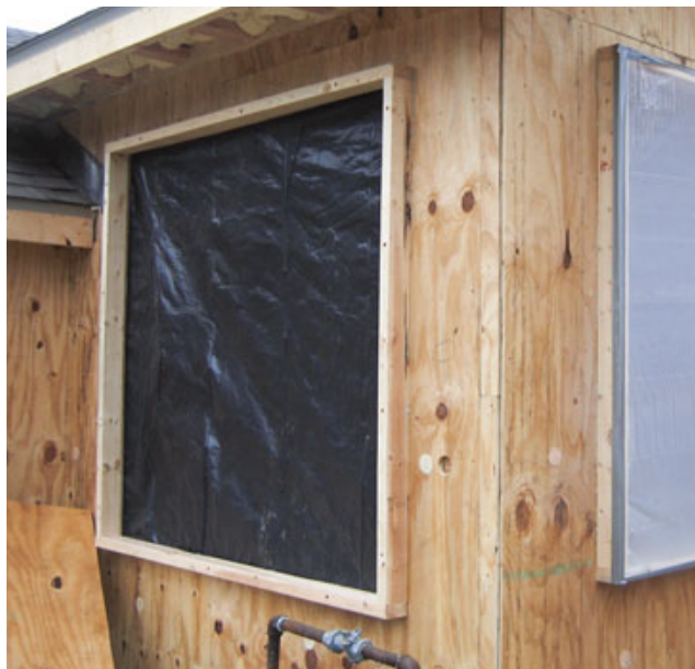
Figure 6. With siding and sheathing removed, potential leaks in the plates were easily sealed with foam (above). Also, as a preventive measure, the exterior bathroom wall was foamed. While nailing up the new sheathing (left), the carpenters took the time to bore holes over each framing cavity — much to the appreciation of the insulation sub who would later fill them with dense-pack cellulose.
