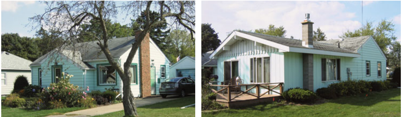
Figure 1. While located in a pleasant residential neighborhood, the original “farmer’s widow house” was drafty and poorly insulated (left). A 1970s addition off the back (right) added much-needed square footage but suffered from the same poor energy performance. In addition to leaving the siding exposed to rain and weather, the absence of eaves overhangs in the front created a visually awkward transition to the broad eaves in the rear.
