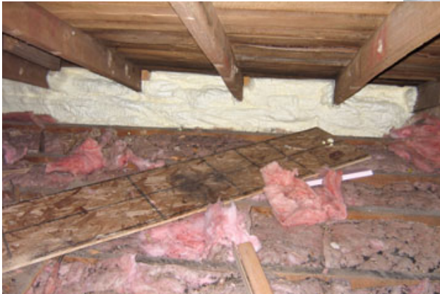
Figure 3. Because the original 2x4 rafters left little space for insulation at the eaves (top left), the area was filled with medium-density spray foam (above), which blocked air leaks and also provided a continuous dam for the cellulose that would be blown into the attic (left). Where excess foam bulged beyond the eaves extensions, the crew cut it away with a sharp handsaw.
