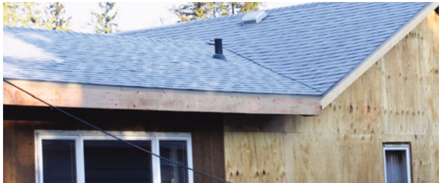
Figure 5. Foil-faced polyiso board, screwed to the addition roof deck (top), supplements the original batts, which were left in place between the rafters. Joints between panels — and the intersection with the board deck of the original house, visible at rear — were sealed with spray foam. The gable-end rake of the original house was extended to meet the addition overhang, providing improved weather protection and a cleaner appearance (right).
