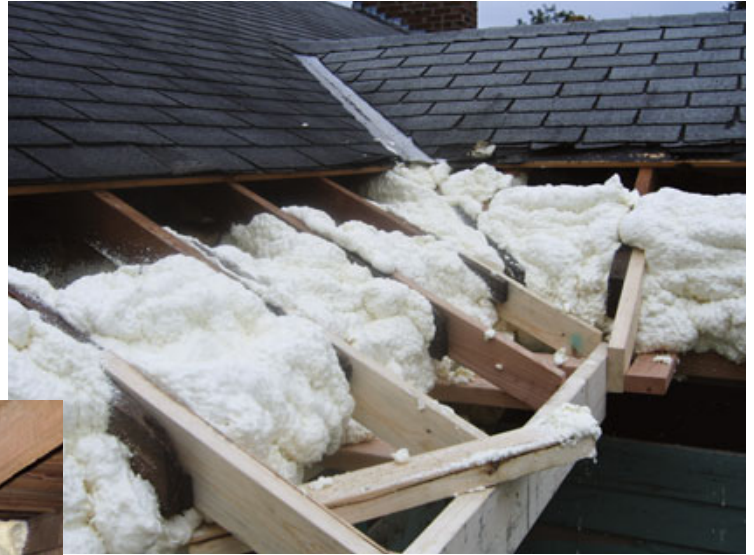
Figure 3. Because the original 2x4 rafters left little space for insulation at the eaves (top left), the area was filled with medium-density spray foam (above), which blocked air leaks and also provided a continuous dam for the cellulose that would be blown into the attic (left). Where excess foam bulged beyond the eaves extensions, the crew cut it away with a sharp handsaw.
