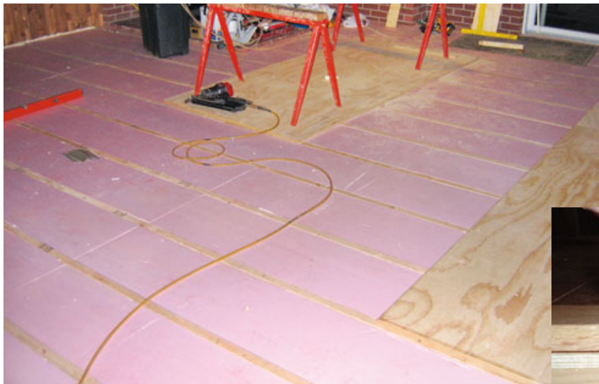
Figure 9. Once stripped of carpeting and tested for moisture, the slab floor of the addition was insulated with XPS foam board fit tightly between lengths of 2-by furring (above). Including the insulation, the finished floor, consisting of \frac{1}{2} -inch plywood and \frac{5}{8} -inch prefinished oak, raised the room's threshold by almost 3 inches (right). A gently sloped transition was added later.
