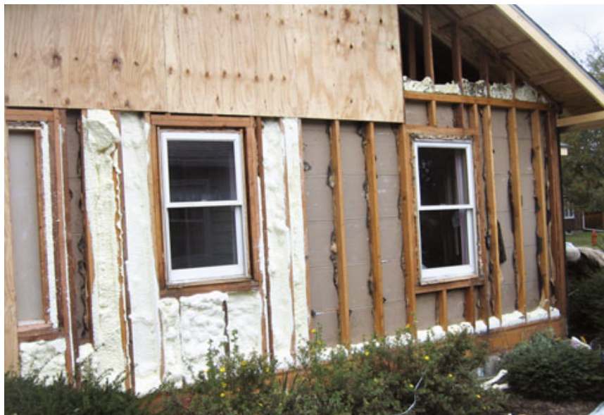
Figure 6. With siding and sheathing removed, potential leaks in the plates were easily sealed with foam (above). Also, as a preventive measure, the exterior bathroom wall was foamed. While nailing up the new sheathing (left), the carpenters took the time to bore holes over each framing cavity — much to the appreciation of the insulation sub who would later fill them with dense-pack cellulose.
