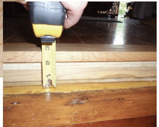
Figure 9. Once stripped of carpeting and tested for moisture, the slab floor of the addition was insulated with XPS foam board fit tightly between lengths of 2-by furring (above). Including the insulation, the finished floor, consisting of \frac{1}{2} -inch plywood and \frac{5}{8} -inch prefinished oak, raised the room's threshold by almost 3 inches (right). A gently sloped transition was added later.
