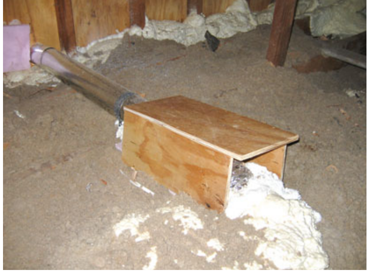
Figure 10. The ERV that supplies the tight retrofitted house with fresh air (above left) is installed at head height in an often-used area, making filter changes easy. The ceiling opening where the flex duct from the new bathroom fan transitions to rigid duct in the attic was enclosed in a plywood box and sprayed with foam for air-sealing and protection from foot traffic (above). The thin, uneven layer of rock wool covering the floor was later covered with 18 inches of loose-fill cellulose. An inexpensive combination thermometer-hygrometer (left) makes it easy to keep an eye on temperature and humidity in several locations, indoor and out.
