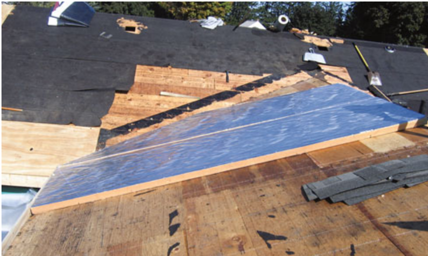
Figure 5. Foil-faced polyiso board, screwed to the addition roof deck (top), supplements the original batts, which were left in place between the rafters. Joints between panels — and the intersection with the board deck of the original house, visible at rear — were sealed with spray foam. The gable-end rake of the original house was extended to meet the addition overhang, providing improved weather protection and a cleaner appearance (right).
