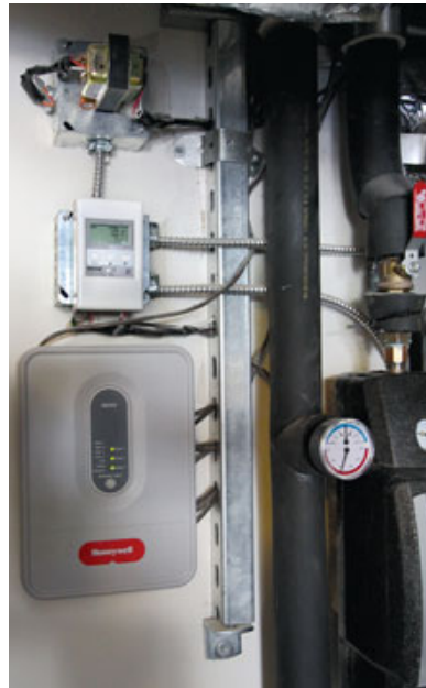
Figure 3. A circulator pumps heat transfer fluid between the storage tank (left) and the solar collectors in response to a set-point control (the white box with the screen, right). The control is programmed to activate the pump when the fluid in the collectors is 15°F hotter than the water in the tank. The gray box beneath the set-point control houses the zone controller, which activates the zone dampers and air handler when a thermostat calls for heat.
