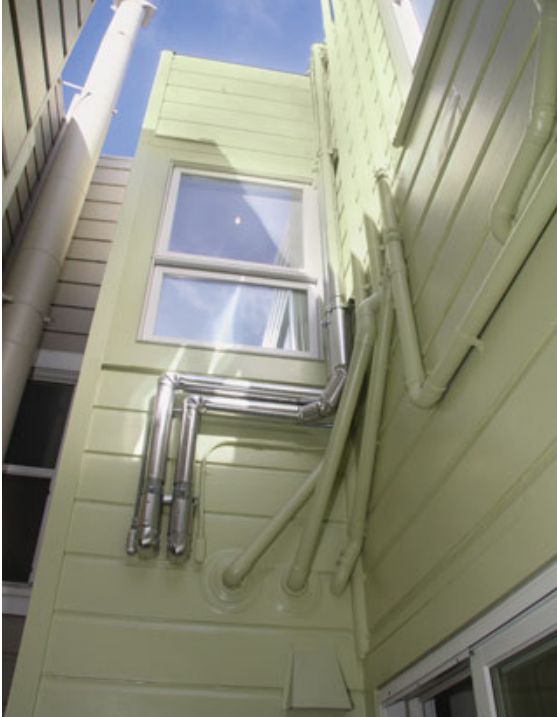
Figure 2. Aluminum cladding protects the insulation on the two pipes that carry fluid to the solar collectors (left). Slightly lower and to the right are the PVC flue and air intake for the condensing boiler. The hood by the door is the HRV's air intake. Further down the wall (above) are the HRV exhaust hood and, to the left of the exhaust, a small pipe that serves as the out-flow for the boiler condensate.
