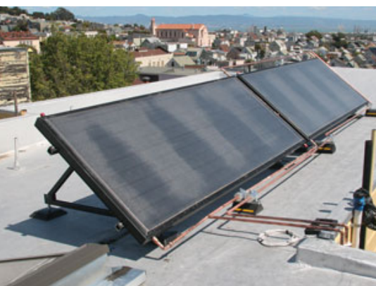
Figure 1. The solar thermal collectors (above) are expected to produce 40 percent of the yearly demand for heat and hot water. The Munchkin boiler (right) will fire whenever the collectors are unable to keep the water in the storage tank at or above 120 degrees.
