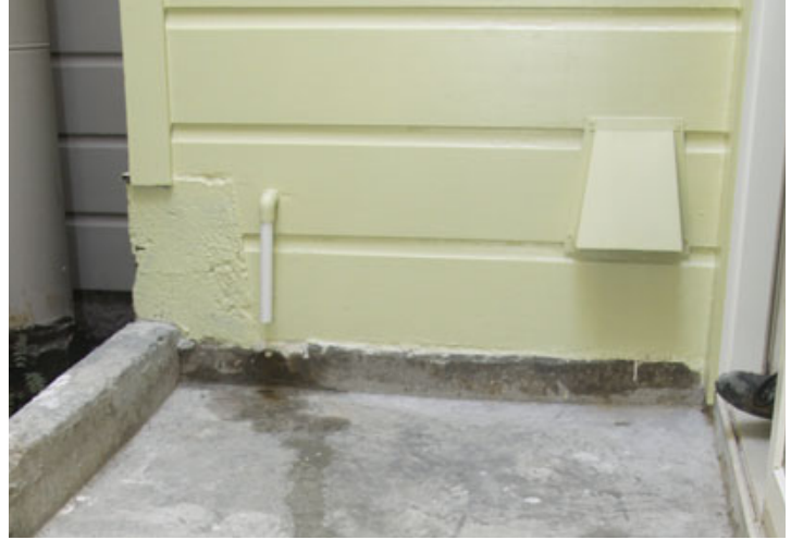
Figure 2. Aluminum cladding protects the insulation on the two pipes that carry fluid to the solar collectors (left). Slightly lower and to the right are the PVC flue and air intake for the condensing boiler. The hood by the door is the HRV's air intake. Further down the wall (above) are the HRV exhaust hood and, to the left of the exhaust, a small pipe that serves as the out-flow for the boiler condensate.
