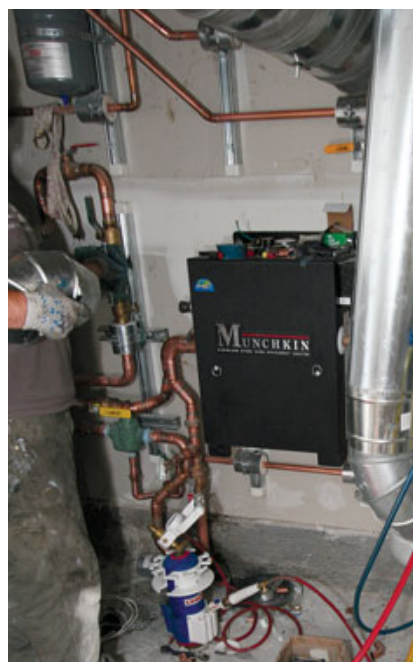
Figure 1. The solar thermal collectors (above) are expected to produce 40 percent of the yearly demand for heat and hot water. The Munchkin boiler (right) will fire whenever the collectors are unable to keep the water in the storage tank at or above 120 degrees.
