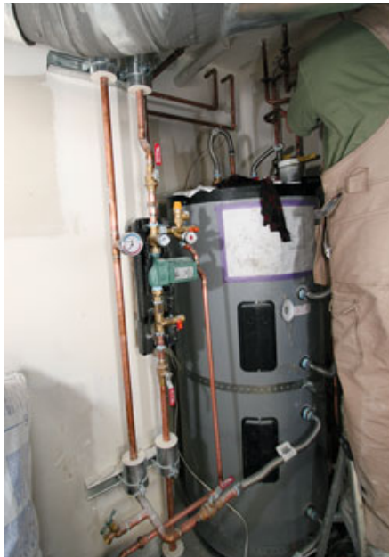
Figure 3. A circulator pumps heat transfer fluid between the storage tank (left) and the solar collectors in response to a set-point control (the white box with the screen, right). The control is programmed to activate the pump when the fluid in the collectors is 15°F hotter than the water in the tank. The gray box beneath the set-point control houses the zone controller, which activates the zone dampers and air handler when a thermostat calls for heat.
