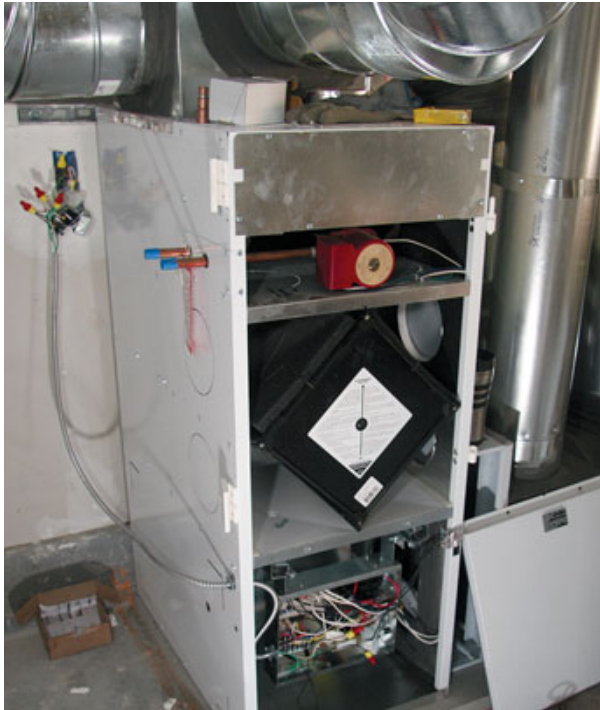
Figure 4. The air handler — a Lifebreath Clean Air Furnace — has a blower below, an HRV in the middle, and a pump and water-to-air heat exchanger coil above. Whenever a thermostat calls for heat, the blower is activated and the pump circulates hot water between the storage tank and the heat exchanger coil. The blower is powered by a high-efficiency motor that modulates between higher speeds in heating mode and low speed when only the HRV is operating.
