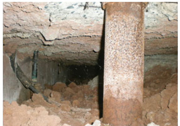
Figure 2. With the drywall stripped from the laundry-room and family-room walls, the sag in both slabs is evident (left). Note the inspection hole in the concrete, which allowed the author to take this photo (right), which shows a large gap between the slab and the soil beneath and, at the back, a disconnected waste line.
