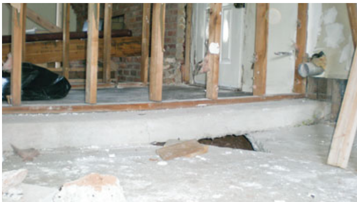
Figure 2. With the drywall stripped from the laundry-room and family-room walls, the sag in both slabs is evident (left). Note the inspection hole in the concrete, which allowed the author to take this photo (right), which shows a large gap between the slab and the soil beneath and, at the back, a disconnected waste line.
