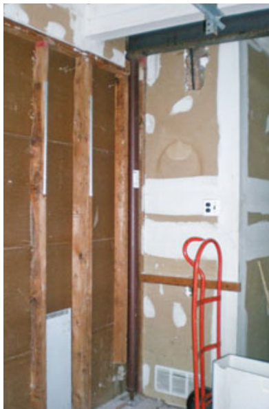
Figure 4. This drywall-covered built-up wood beam (top) was offset 2 feet from the front eaves wall it was meant to support. To correct the faulty load path, a new steel I-beam, supported by steel posts at each end (right), was installed in the correct place. A new footing was poured for a steel post at midspan (above).
