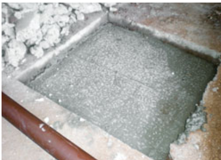
Figure 4. This drywall-covered built-up wood beam (top) was offset 2 feet from the front eaves wall it was meant to support. To correct the faulty load path, a new steel I-beam, supported by steel posts at each end (right), was installed in the correct place. A new footing was poured for a steel post at midspan (above).
