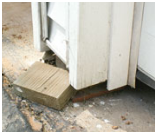
Figure 1. Careless site preparation at the time of construction left this 30-year-old home with a sinking driveway, a cracked and leaking sewer line, and failed slabs in the garage and the family room behind it (top). The gap beneath the garage door (above left and left) was a full 8 inches high at the right-hand side. At the back of the garage, the laundry-room wall was separating from the slab (above).
