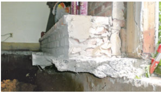
Figure 6. With the second-story loads permanently supported, slab demolition (above left) and excavation (above) could take place. Because the exterior framing sat on top of the slab, it was simpler to cut the concrete cleanly at the inside edge of the perimeter wall. The weight of the brickwork above the family room hearth (left) proved sufficient to hold the hearth extension in place until new support walls could be provided in the crawlspace below.
