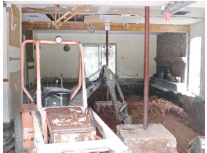
Figure 6. With the second-story loads permanently supported, slab demolition (above left) and excavation (above) could take place. Because the exterior framing sat on top of the slab, it was simpler to cut the concrete cleanly at the inside edge of the perimeter wall. The weight of the brickwork above the family room hearth (left) proved sufficient to hold the hearth extension in place until new support walls could be provided in the crawlspace below.
