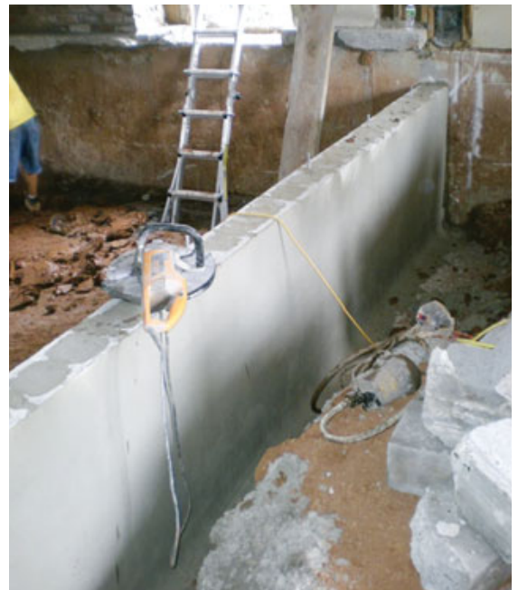
Figure 7. A new steel-reinforced footing, anchored to holes drilled in the existing perimeter wall (above left) supports a block foundation wall between the laundry room and garage (above). An access opening between the new crawlspace and the existing basement (left) was cut with a concrete saw equipped with a diamond blade. Note the sump cover.
