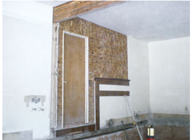
Figure 3. To prevent demolition dust from spilling into the living space beyond (left), the contractor built a temporary wall with a passage door (right).
