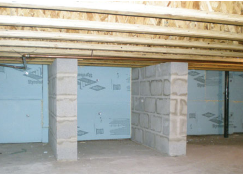
Figure 8. The existing hearth extension gained additional support from a pair of short block walls and the short steel column visible at far right of photo (above). The column's upper end was tightened against the cantilevered section of slab; a few squirts of polyurethane foam prevent squeaks between the slab and the OSB floor sheathing (above right). After the new laundry and family-room floor was framed and sheathed, the garage area was backfilled with compacted gravel in preparation for the new slab (right).
