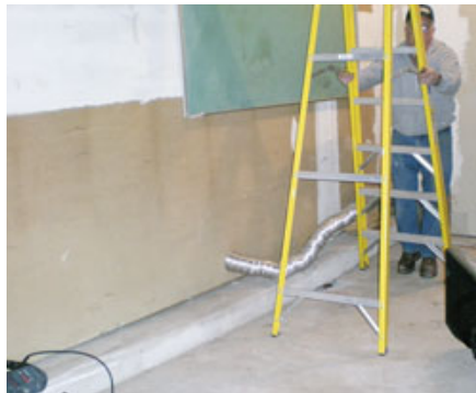
Figure 1. Careless site preparation at the time of construction left this 30-year-old home with a sinking driveway, a cracked and leaking sewer line, and failed slabs in the garage and the family room behind it (top). The gap beneath the garage door (above left and left) was a full 8 inches high at the right-hand side. At the back of the garage, the laundry-room wall was separating from the slab (above).
