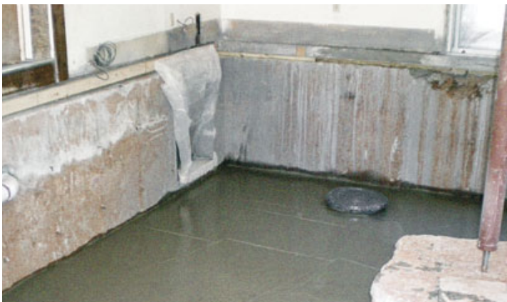
Figure 7. A new steel-reinforced footing, anchored to holes drilled in the existing perimeter wall (above left) supports a block foundation wall between the laundry room and garage (above). An access opening between the new crawlspace and the existing basement (left) was cut with a concrete saw equipped with a diamond blade. Note the sump cover.
