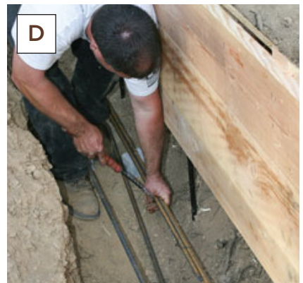
Figure 4. The retaining wall foundation required a serious amount of rebar, including L-shaped pieces coming up from a wide footing (A), tied in a 12-inch grid to the top of the wall (B). To speed tying and ease wrist strain, the crew used inexpensive manual twist tools that wind the ends of the wire when their handle is pulled (C, D). The author rented a heavy-duty electric bender to speed the work (E).
