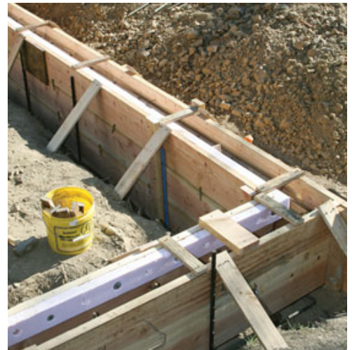
Figure 7. For stem walls, the author uses 2x10s with form ties that also support rebar (above left). Where the patio and garage slabs were to be poured, the crew lined the inside form with a strip of rigid foam to create a ledge for the slab (above). L-shaped rebar elbows inserted through the form horizontally (left) will allow the eventual grid of rebar in the slab to be tied to the rebar in the perimeter stem wall.
