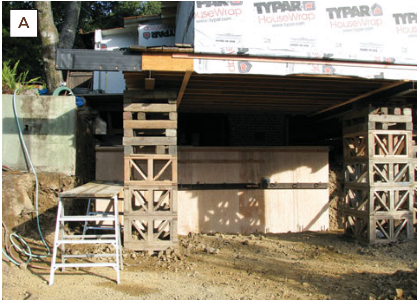
Figure 3. The plans called for extensive digging under the house. To avoid undermining the existing fireplace, which was to be left in place, the crew installed temporary plywood shoring pinned to the earth with heavy rebar (A, B). This created a safe though narrow work space for forming and pouring a new retaining wall (C). The new reinforced wall would serve as the back wall of the downstairs living space and permanently stabilize the soil under the house (D).
