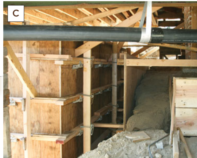
Figure 3. The plans called for extensive digging under the house. To avoid undermining the existing fireplace, which was to be left in place, the crew installed temporary plywood shoring pinned to the earth with heavy rebar (A, B). This created a safe though narrow work space for forming and pouring a new retaining wall (C). The new reinforced wall would serve as the back wall of the downstairs living space and permanently stabilize the soil under the house (D).
