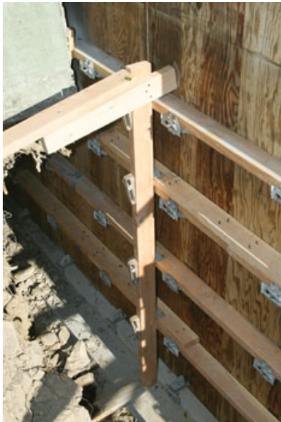
Figure 5. Concrete is pumped into one of the new basement walls (top). The author uses a simple forming system from Meadow Burke that includes durable reusable hardware for attaching snap-ties, walers, and upright braces (above left). The waler system is designed for use with plywood, which is predrilled in stacks to match the snap-tie layout (above right).
