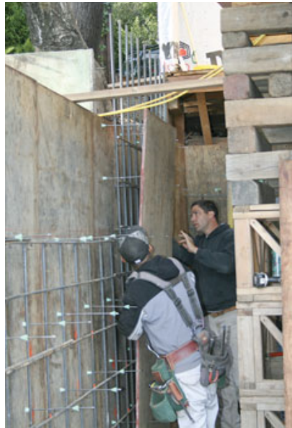
Figure 5. Concrete is pumped into one of the new basement walls (top). The author uses a simple forming system from Meadow Burke that includes durable reusable hardware for attaching snap-ties, walers, and upright braces (above left). The waler system is designed for use with plywood, which is predrilled in stacks to match the snap-tie layout (above right).
