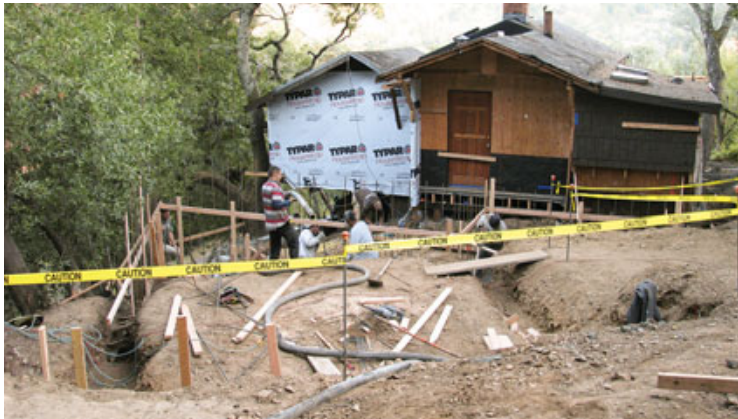
Figure 1. Perched on a hillside with a fantastic view, the former hunting camp was in a prime location. But structural details like the original post foundation, dating back to the mid-1930s, fell far short of California’s modern code requirements for seismic engineering. At left, the view from the driveway, where the new garage foundation is being laid out.
