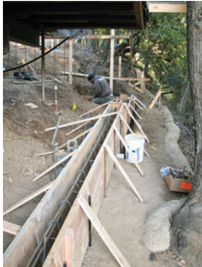
Figure 6. Where the roots of old oak trees grew under the house, the crew stopped trenching (left, center) and instead formed engineered grade beams to connect the discontinued footings in those locations. The tree roots continue to grow undisturbed beneath the grade beams (right).
