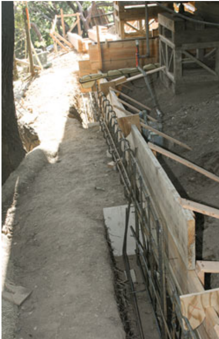
Figure 6. Where the roots of old oak trees grew under the house, the crew stopped trenching (left, center) and instead formed engineered grade beams to connect the discontinued footings in those locations. The tree roots continue to grow undisturbed beneath the grade beams (right).
