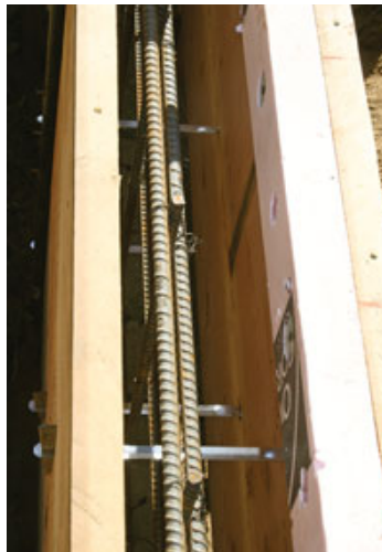
Figure 6. Where the roots of old oak trees grew under the house, the crew stopped trenching (left, center) and instead formed engineered grade beams to connect the discontinued footings in those locations. The tree roots continue to grow undisturbed beneath the grade beams (right).
