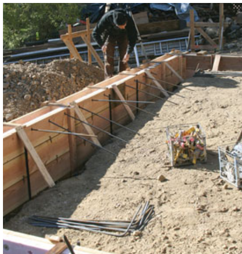
Figure 7. For stem walls, the author uses 2x10s with form ties that also support rebar (above left). Where the patio and garage slabs were to be poured, the crew lined the inside form with a strip of rigid foam to create a ledge for the slab (above). L-shaped rebar elbows inserted through the form horizontally (left) will allow the eventual grid of rebar in the slab to be tied to the rebar in the perimeter stem wall.
