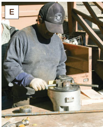
Figure 4. The retaining wall foundation required a serious amount of rebar, including L-shaped pieces coming up from a wide footing (A), tied in a 12-inch grid to the top of the wall (B). To speed tying and ease wrist strain, the crew used inexpensive manual twist tools that wind the ends of the wire when their handle is pulled (C, D). The author rented a heavy-duty electric bender to speed the work (E).
