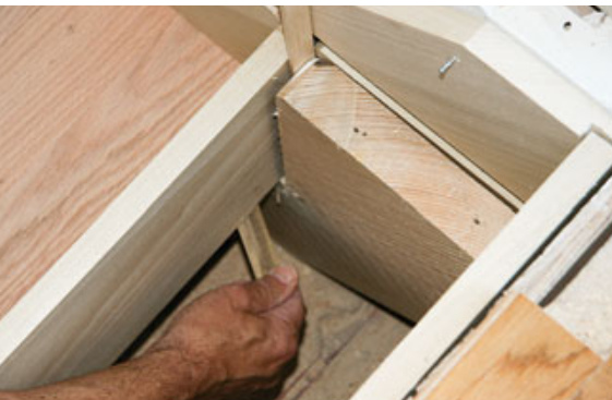
Figure 5. Routs in the skirtboards are cut to allow the treads and risers to be deeply inserted on one side, then withdrawn halfway to engage the opposite, shallower skirt (above photos). Treads and risers are inserted into the left-hand skirtboard first (left, top), then slid back to seat in the right-hand side (left, center). Shimming under the tread snugs it tight against the housing; construction adhesive permanently fills the unseen gaps (left, bottom). A slight block-planed bevel on leading tread corners helps ease the tilt-in installation (illustration).
