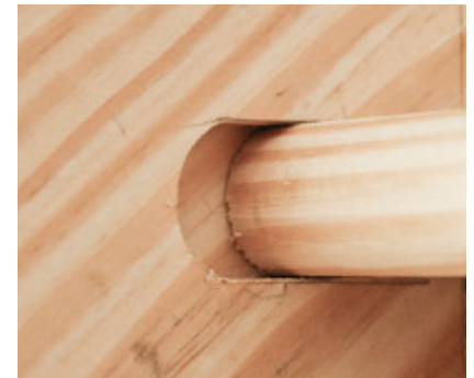
Figure 5. Routs in the skirtboards are cut to allow the treads and risers to be deeply inserted on one side, then withdrawn halfway to engage the opposite, shallower skirt (above photos). Treads and risers are inserted into the left-hand skirtboard first (left, top), then slid back to seat in the right-hand side (left, center). Shimming under the tread snugs it tight against the housing; construction adhesive permanently fills the unseen gaps (left, bottom). A slight block-planed bevel on leading tread corners helps ease the tilt-in installation (illustration).
