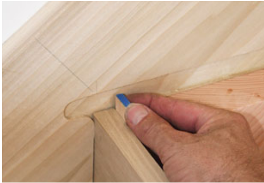
Figure 6. On the lower treads, a glued shim fills the gap between the riser and stringer, snugging the riser tight in the housing. Because the landing nosing is already in place, temporary screws are used to push the topmost riser back onto the tread. When the adhesive sets up, they're removed and the holes are repaired.
