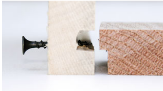
Figure 2. A glued, interlocking joint between tread and riser eliminates movement and friction squeaks. Screws inserted beneath the tongue force the tread slightly upward, making a tight-looking joint.
