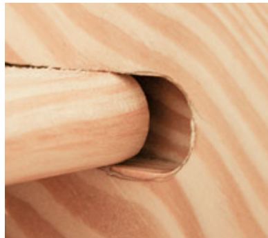
Figure 5. Routs in the skirtboards are cut to allow the treads and risers to be deeply inserted on one side, then withdrawn halfway to engage the opposite, shallower skirt (above photos). Treads and risers are inserted into the left-hand skirtboard first (left, top), then slid back to seat in the right-hand side (left, center). Shimming under the tread snugs it tight against the housing; construction adhesive permanently fills the unseen gaps (left, bottom). A slight block-planed bevel on leading tread corners helps ease the tilt-in installation (illustration).
