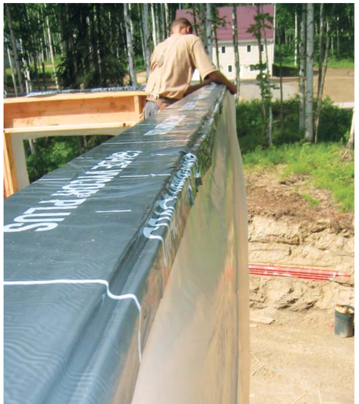
Figure 2. The author's crew applies a 9-inch-wide peel-and-stick flashing to the top plates, adhering it to the inside edge of the plates (top) and lapping it onto the 6-mil poly membrane on the sheathing (above).
