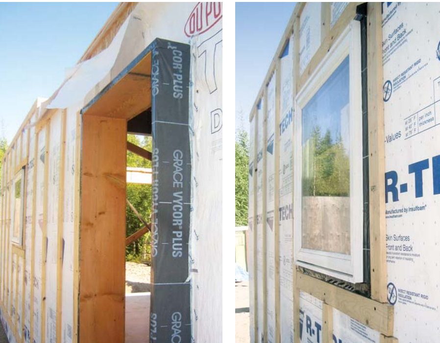
Figure 4. On past jobs, the author installed windows at the face of the wall by setting them in solid lumber bucks protected with peel-and-stick flashing (top). The bucks are attached to the inside of the rough opening and taped or flashed to the wall membrane (above left). Bucks are sized so that when foam insulation and furring are installed, the siding will be in the proper plane (above right).
