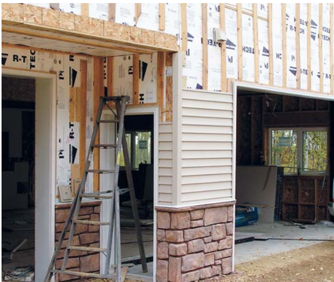
Figure 6. The EPS insulation is first tacked in place, then secured with long screws fastened through furring strips into the framing (top left). Wide furring members are needed at corners (top right) and around openings (above) to provide backing for trim.
