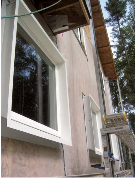
Figure 3. When installing recessed windows, the author uses sill and jamb extensions bent from coated sheet metal. The flanges at the outer edges (left) are carefully placed to allow for the thickness of the foam, \frac{3}{4} -inch strapping, and the vinyl siding, which will tuck underneath. Note the lines of black acoustical caulk used to seal the jamb extensions to the poly membrane and the poly seams (above).
