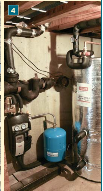
Photos 1, 2, and 4: Michael Morris; Photo 3: Alchemy Construction
