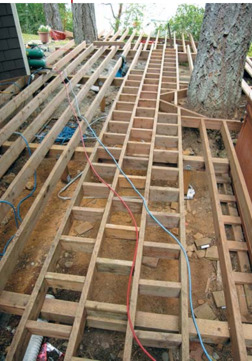
Figure 3. Blocking parallel to the joists for the long inlay on the upper deck was relatively simple (above left), but blocking the curved section on the lower deck took a lot of layout and numerous individually cut pieces (above right).
