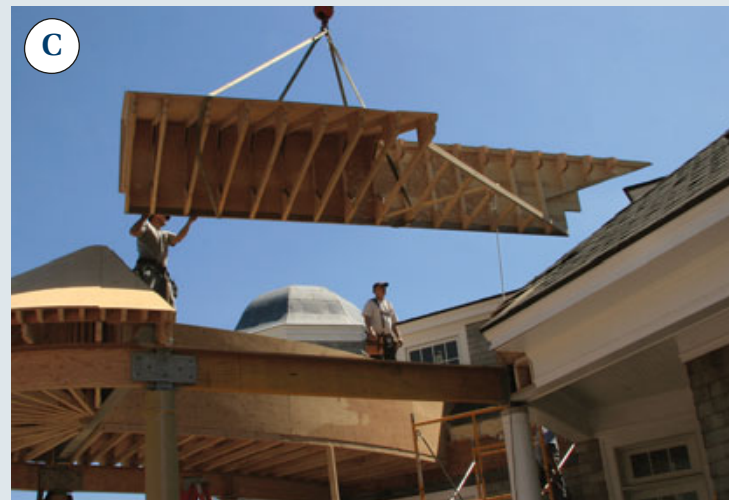
Figure 1. The roof framing consists of five modules assembled on site, beginning with the half cone (A). The four major modules all bear on the perimeter architrave beam and a steel moment frame at the cone's midsection. The fifth, nonstructural module (E) completes the top and back of the cone.
