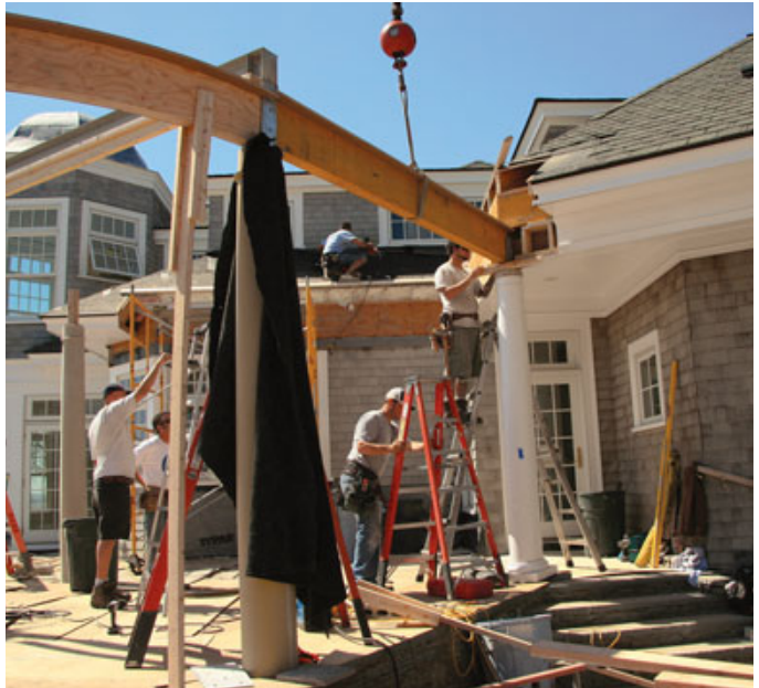
Figure 8. The architrave is supported on 4x6 pressure-treated posts within the architectural columns, notched to 4x4s where they pass through the beam (above left). The only straight section in the architrave is made with doubled LVL lumber (above). Welded brackets support the beam at the moment frame (left).
