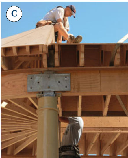
Figure 9. While the welder put the finishing touches on the moment frame, the crew set the roof modules around the architrave (A). Each module included a recess to encase and bear upon the moment beam (B). Metal plates tie the architrave to the steel posts (C); wood post locations were tied together with plywood overlays. A slight built-in tolerance allowed the center module to drop in without resistance (D). The "bat" module defines the valleys and completes the cone (E).
