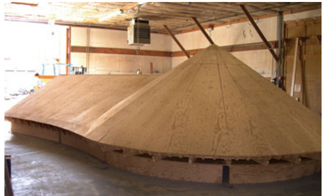
Figure 7. The center roof module fills the progressively widening space between the side modules (left). Hold-offs, back-screwed to the upright truss members, reserve the space that will be occupied by five layers of plywood once the center module is framed and pulled free for access (below left). With the sheathing and cap completed, the modules were ready for transport to the job site (below).
