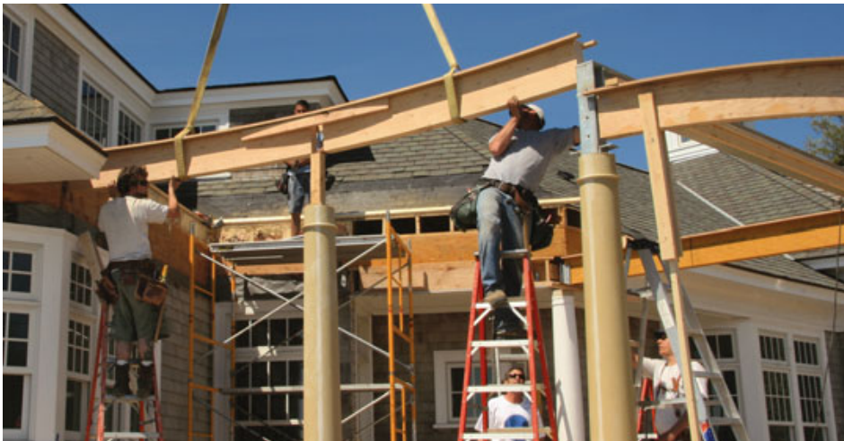
Figure 8. The architrave is supported on 4x6 pressure-treated posts within the architectural columns, notched to 4x4s where they pass through the beam (above left). The only straight section in the architrave is made with doubled LVL lumber (above). Welded brackets support the beam at the moment frame (left).
