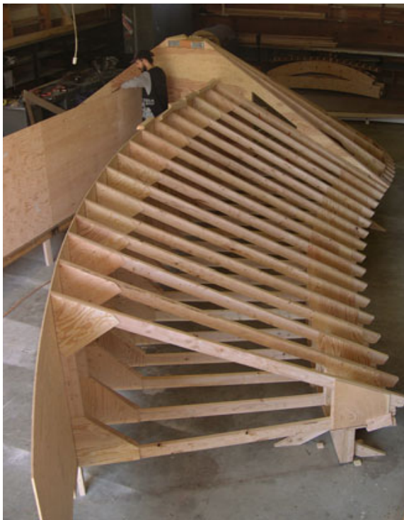
Figure 5. A worker installs bevel-edged blocking between the trusses to provide nailing for the roof sheathing at the top edge, where the roof line transitions to a flat midsection. Here, the trusses have received the first of five layers of \frac{3}{8} -inch UL plywood, forming a structural beam that supports the center module.
