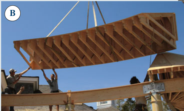
Figure 1. The roof framing consists of five modules assembled on site, beginning with the half cone (A). The four major modules all bear on the perimeter architrave beam and a steel moment frame at the cone's midsection. The fifth, nonstructural module (E) completes the top and back of the cone.
