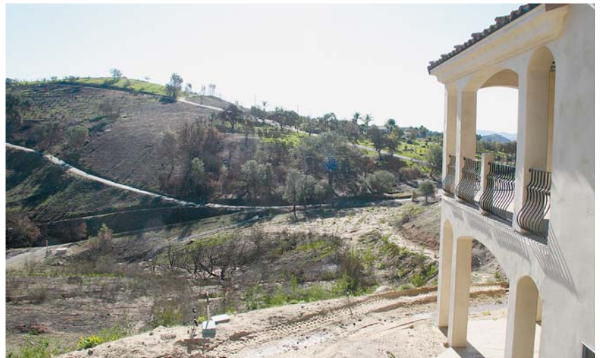
Figure 6. This Ranch Santa Fe deck (above) complies with ignition-resistant requirements because of its heavy timber framing, nominal 2x6 planking, and metal support posts and railing system. The deck at top right, stuccoed on the underside and topped with a proprietary noncombustible polymer waterproofing, also meets the code. Another view of that deck (right) shows the blackened hillside and recent green growth where the October fire swept around two sides of the house, leaving the structure undamaged.
