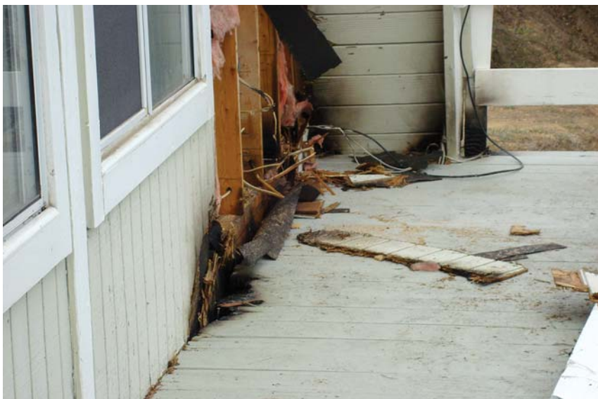
Figure 5. Combustible deck structures are a critical vulnerability in wildfire country. Here, windblown embers collected at the intersection of a wood deck and wall during October's fire, igniting the house exterior.
