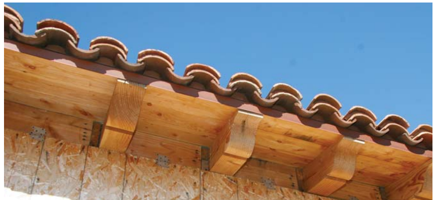
Figure 3. The photo above shows an eave with wire reinforcement in place, ready for stucco application. The completed eave (above right) presents the appearance of solid masonry. At right, metal clips connect the wood structural panel sheathing to the blocking between rafters, a required seismic detail in Southern California.
