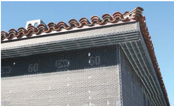
Figure 3. The photo above shows an eave with wire reinforcement in place, ready for stucco application. The completed eave (above right) presents the appearance of solid masonry. At right, metal clips connect the wood structural panel sheathing to the blocking between rafters, a required seismic detail in Southern California.
