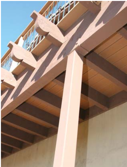
Figure 6. This Ranch Santa Fe deck (above) complies with ignition-resistant requirements because of its heavy timber framing, nominal 2x6 planking, and metal support posts and railing system. The deck at top right, stuccoed on the underside and topped with a proprietary noncombustible polymer waterproofing, also meets the code. Another view of that deck (right) shows the blackened hillside and recent green growth where the October fire swept around two sides of the house, leaving the structure undamaged.
