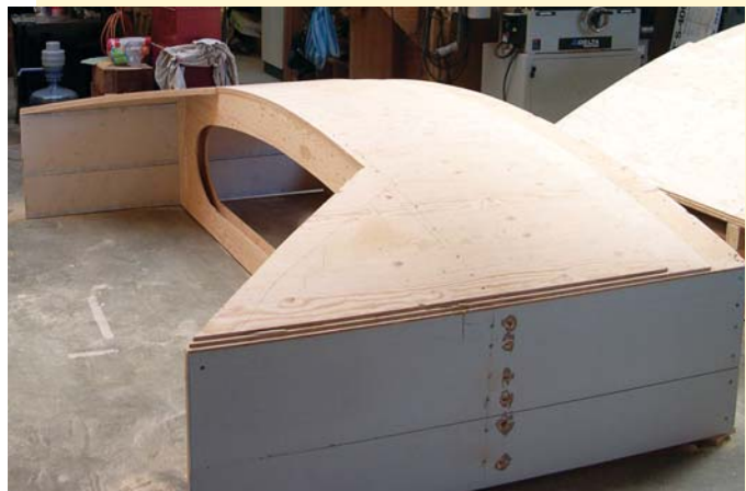
Figure 3. The roof was made in two pieces, a front rectangular section (top) and a rear section (above) cut out to wrap a projecting bay. The sheathing was applied in three layers, stepped back at the joint between the sections to allow for a strong overlapping layer of sheathing to be applied on site. The small overhang across the front of the roof (left), made from cedar, was blended at the corners with a filler of epoxy and sawdust, then sanded flush.
