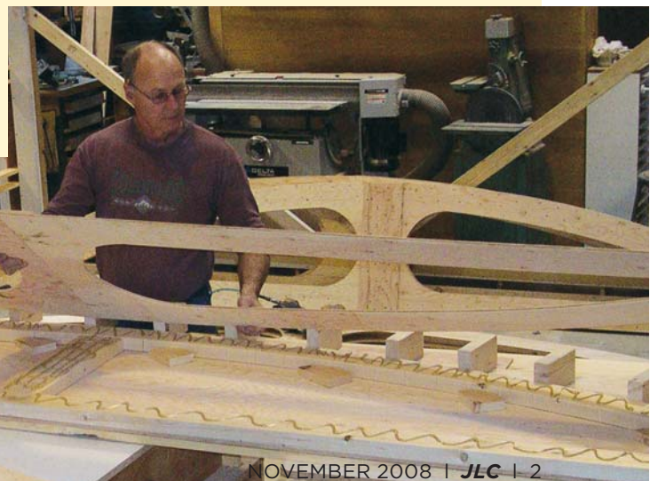
Figure 2. The arch-topped roof trusses are made from 2x4 chords skinned with \frac{3}{8} -inch plywood. To form a graceful curve, the author bent a flexible piece of pine between the roof's rise and run and traced the profile onto the plywood (above). The first half-rafter was carefully cut out, then used as a pattern for the others (above right). The plywood cutouts were joined end to end with plywood plates, then glued and stapled to both sides of the framing members, creating strong, lightweight trusses 16 feet long (bottom).
