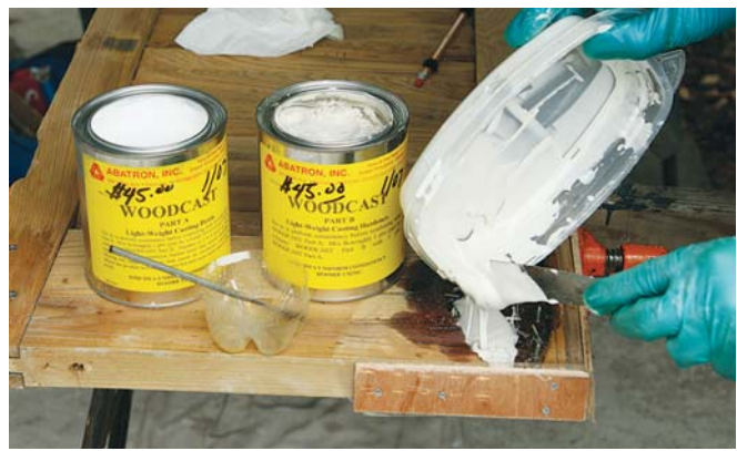
Figure 3. After using a rotary rasp and a variety of hand picks to remove rotted wood (top left), the author fills the depression with epoxy-based products, starting with LiquidWood consolidant (top right) and following with WoodEpoxy compound (above left). Abatron's Woodcast, applied against the plywood form, helps shape the new corner (above). West Systems epoxy, thickened with chopped fiberglass, provides bulk (far left), and is followed by another light coat of WoodEpoxy to make final sanding easier (left).
