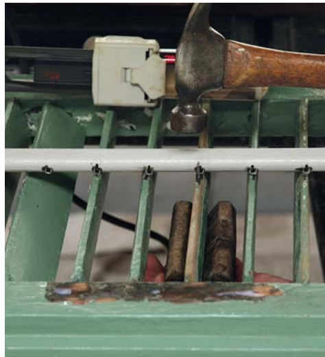
Figure 6. Occasionally it's necessary to make a new control rod. After drilling holes for the staples, the author puts a dab of glue in the holes (above left), then drives each staple home (above). He repeats the process when linking the rod staples to the slat staples (far left and left).
