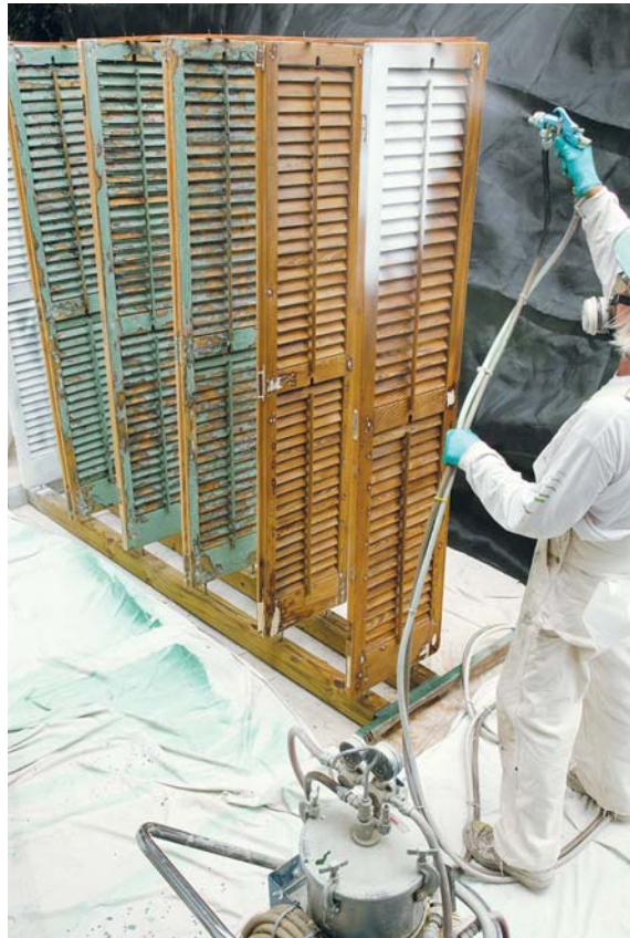
Figure 7. With a 25-foot hose and a remote pressure pot, the author's spray rig allows him plenty of mobility to get in between the shutters on the spray rack. After all the coats have been applied, he fills the holes in the bottoms of the shutters and coats tops and bottoms with a brush.
