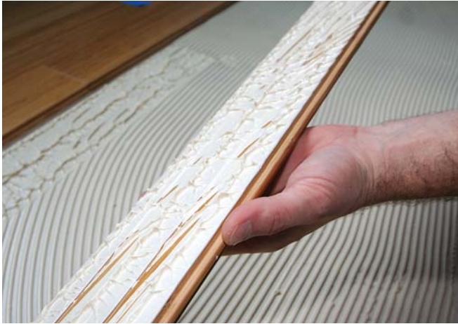
Figure 5. To make certain he is applying enough adhesive, the author occasionally pulls up a piece of flooring to check the coverage (left). Because flooring can slide around on the wet adhesive, he uses painter’s tape to hold the edge and end joints tight until the glue dries (below). Squeeze-out is wiped clean with a damp rag (bottom).
