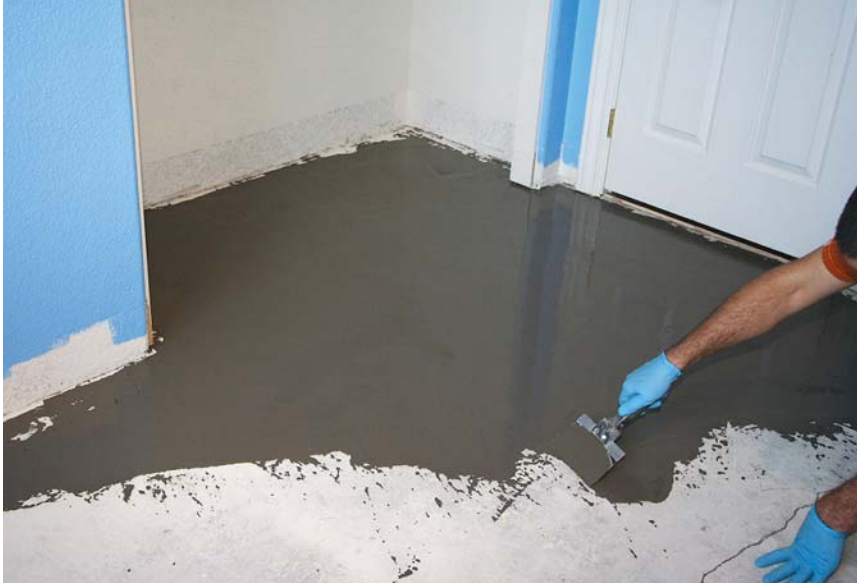
Figure 2. Slab flatness should be within \frac{3}{16} inch over 10 feet. High spots can be ground down when necessary; low spots are filled with a leveling compound (above). After flattening the floor, the author uses a Fein MultiMaster (right) to trim jambs and casings so the flooring will slip underneath.
