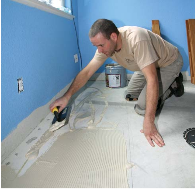
Figure 4. The author spreads adhesive to a line traced on the floor (above), then beds the first course of flooring, placing shims that position it exactly parallel to layout (right). Successive courses are laid exactly as they were positioned when dry-fit (below).
