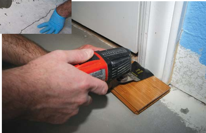
Figure 2. Slab flatness should be within \frac{3}{16} inch over 10 feet. High spots can be ground down when necessary; low spots are filled with a leveling compound (above). After flattening the floor, the author uses a Fein MultiMaster (right) to trim jambs and casings so the flooring will slip underneath.
