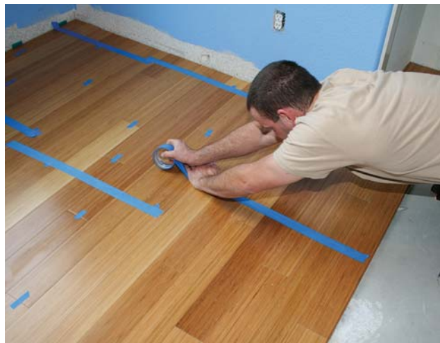
Figure 5. To make certain he is applying enough adhesive, the author occasionally pulls up a piece of flooring to check the coverage (left). Because flooring can slide around on the wet adhesive, he uses painter’s tape to hold the edge and end joints tight until the glue dries (below). Squeeze-out is wiped clean with a damp rag (bottom).
