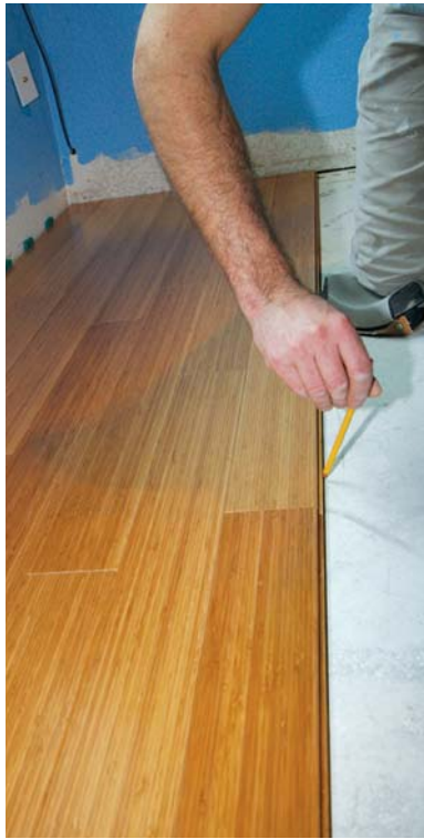
Figure 3. With the first course shimmed to a layout line, the author starts dry-fitting the flooring (far left), creating a random stagger by using starting pieces of varying length. He traces an edge every couple of feet to mark how far to spread adhesive as he works a section at a time (left). He checks layout as he goes (below) and, after racking the entire floor, stages the pieces neatly (bottom) so that they go back down in the same order over the wet adhesive.
