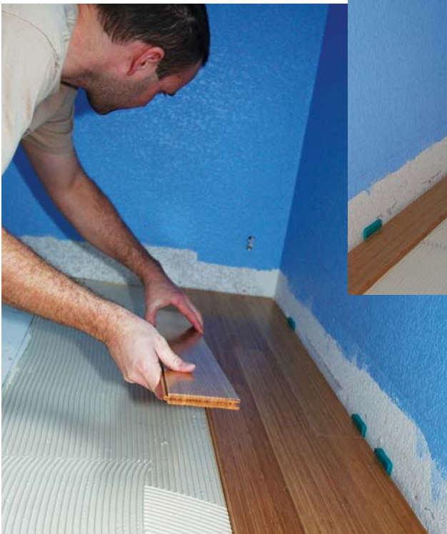
Figure 4. The author spreads adhesive to a line traced on the floor (above), then beds the first course of flooring, placing shims that position it exactly parallel to layout (right). Successive courses are laid exactly as they were positioned when dry-fit (below).
