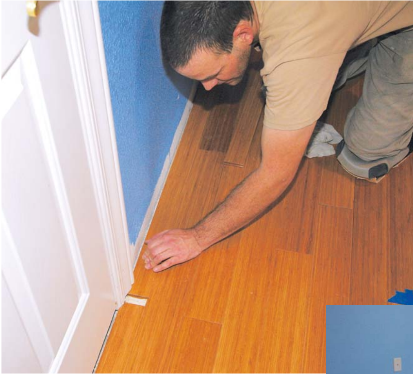
Figure 6. Careful layout ensures that the last piece of flooring is the same width as the first and can be slipped into place under the door casing (left). Below, the finished floor.
