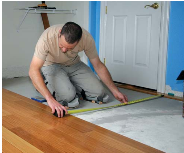
Figure 3. With the first course shimmed to a layout line, the author starts dry-fitting the flooring (far left), creating a random stagger by using starting pieces of varying length. He traces an edge every couple of feet to mark how far to spread adhesive as he works a section at a time (left). He checks layout as he goes (below) and, after racking the entire floor, stages the pieces neatly (bottom) so that they go back down in the same order over the wet adhesive.
