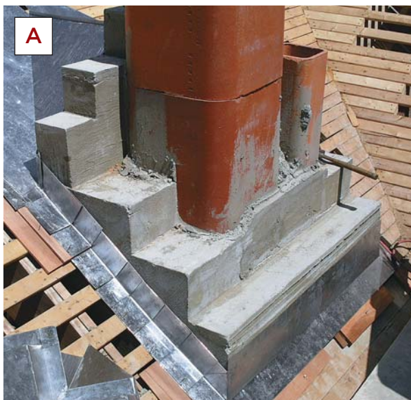
Figure 4. The base flashings — including the step flashings and front apron (A) and the cricket (B) — are installed first. The two-piece cricket is made in the shop — using a brake to ensure straight valley creases — then brought to the roof, where the ridge seam is bent in place with a hand seamer and a rawhide mallet.
