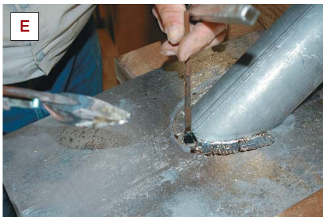
Figure 1. Before soldering, author John Seifert tins the copper tip: He rubs it on a soft brick to clean it (A) and then on a block of sal ammoniac (B), a soft mineral that provides an oxide-free zone around the heated tip, thereby allowing the solder to coat it. Here, working on a vent-stack shroud, he first applies enough solder to connect the joint (C), then goes back and applies a heavier layer of solder (D) to fill possible pinholes. Flux, applied before and during the process (E), cleans the metal and helps the solder flow.
