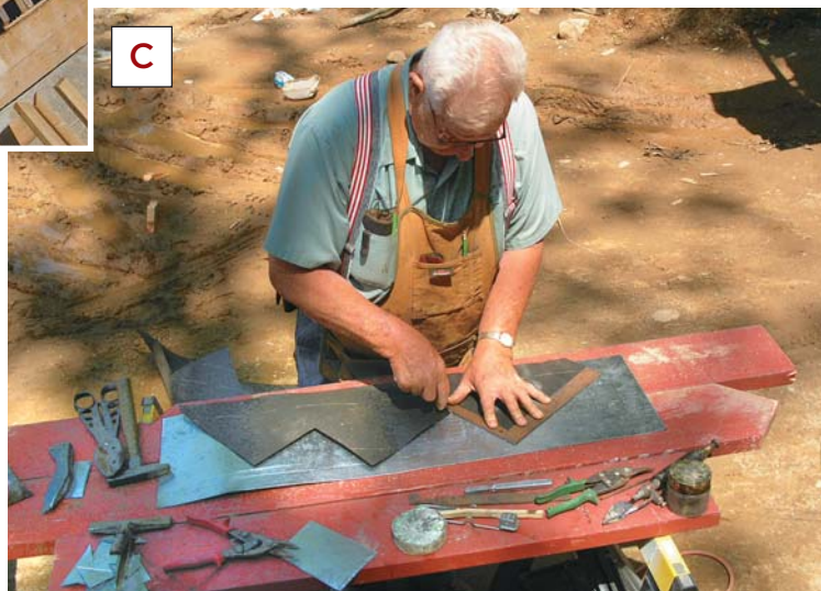
Figure 2. Working directly from the masonry base (A), John traces a template of the stepped shoulders (B), which co-author Fred Seifert uses to cut the side flashings (C).
