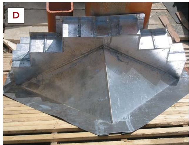
Figure 5. Counterflashings cover the base flashings but are not soldered to them, so that the masonry can move separately from the roof structure without creating a leak. Here, Fred fits the apron counterflashing (A) and — with the corner seam temporarily clamped in place — solders it to the top of stepped side flashing (B). The vertical corner seams will then be folded, tightened with a mallet, and soldered. Weep channels, soldered on top of the steps (C, D), complete the job.
