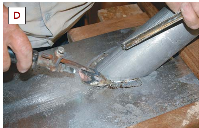
Figure 1. Before soldering, author John Seifert tins the copper tip: He rubs it on a soft brick to clean it (A) and then on a block of sal ammoniac (B), a soft mineral that provides an oxide-free zone around the heated tip, thereby allowing the solder to coat it. Here, working on a vent-stack shroud, he first applies enough solder to connect the joint (C), then goes back and applies a heavier layer of solder (D) to fill possible pinholes. Flux, applied before and during the process (E), cleans the metal and helps the solder flow.
