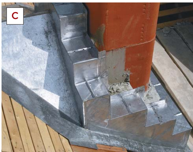
Figure 5. Counterflashings cover the base flashings but are not soldered to them, so that the masonry can move separately from the roof structure without creating a leak. Here, Fred fits the apron counterflashing (A) and — with the corner seam temporarily clamped in place — solders it to the top of stepped side flashing (B). The vertical corner seams will then be folded, tightened with a mallet, and soldered. Weep channels, soldered on top of the steps (C, D), complete the job.
