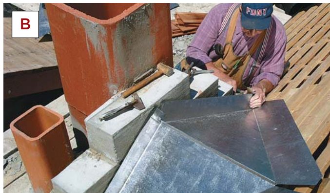
Figure 4. The base flashings — including the step flashings and front apron (A) and the cricket (B) — are installed first. The two-piece cricket is made in the shop — using a brake to ensure straight valley creases — then brought to the roof, where the ridge seam is bent in place with a hand seamer and a rawhide mallet.
