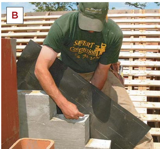
Figure 2. Working directly from the masonry base (A), John traces a template of the stepped shoulders (B), which co-author Fred Seifert uses to cut the side flashings (C).
