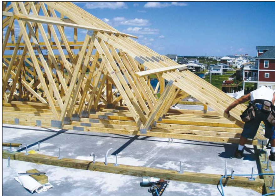
FIGURE 7. Pitched truss roofs for the concrete houses are set on treated-wood beams anchored to the flat top of the concrete box. Mechanicals can be installed in the attic if need be, and attic floors can receive deep blown fiber insulation for an airtight, highly insulated lid. Damage to the roof structure during a severe windstorm does not compromise the structural integrity of the rest of the building.
