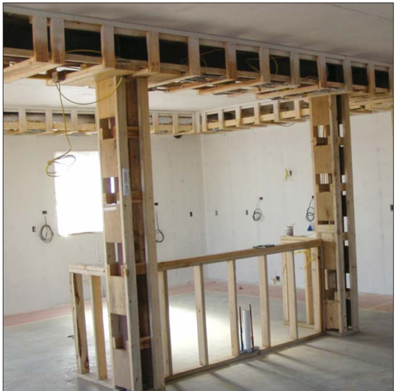
FIGURE 8. Red-iron beams (top) allow the creation of larger open spaces inside the houses. Wood-framed chases (above) can be used for architectural detail and to hide steel or ductwork. Plaster or drywall compound (left) applied directly to the concrete walls leaves the thermal mass of the concrete in contact with the occupied space.
