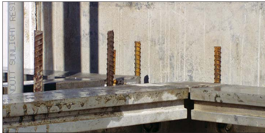
FIGURE 5. Special ledger cap forms are clipped to the top of the inside wall forms (above). Shoring beams of various lengths and widths integrate with the slab forms to allow for a range of floor sizes (left). Crews set slab form panels to span between the ledger forms and the shoring beams (below), creating the form system for a monolithic wall-and-slab pour.
