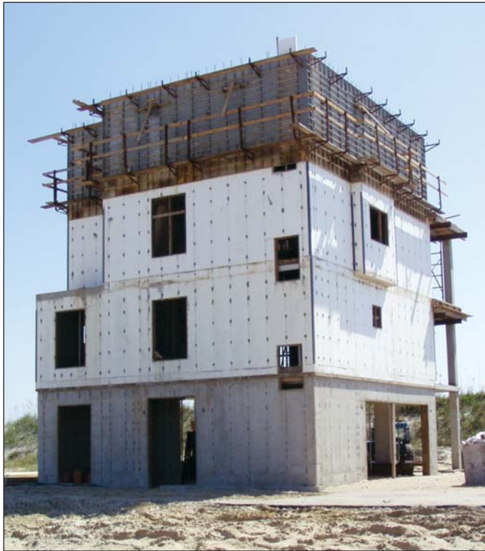
FIGURE 2. After the first elevated slab is set, crews can add as many as three more occupied stories in successive monolithic pours using the Wall Ties aluminum form system (left). Note the foam insulation (still exposed at this stage), which is placed against exterior forms before the pour and remains in place after forms are stripped. Pitched roofs are framed as a wood truss structure, on top of the main flat-topped concrete box (below).
