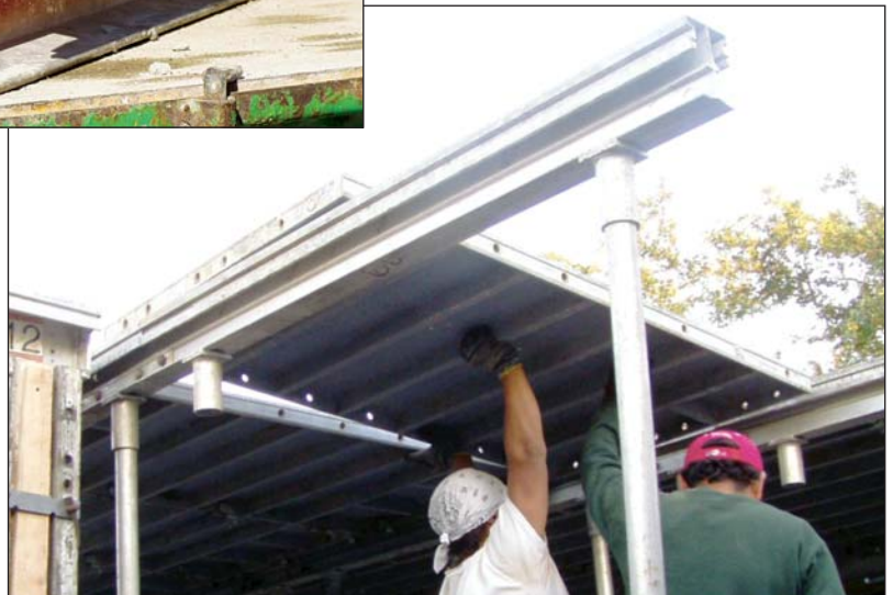
FIGURE 5. Special ledger cap forms are clipped to the top of the inside wall forms (above). Shoring beams of various lengths and widths integrate with the slab forms to allow for a range of floor sizes (left). Crews set slab form panels to span between the ledger forms and the shoring beams (below), creating the form system for a monolithic wall-and-slab pour.
