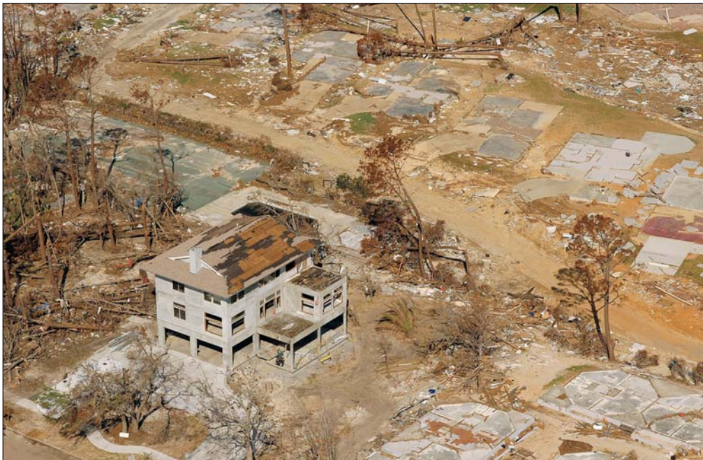
FIGURE 1. This poured-concrete house in Pass Christian, Miss., survived the storm surge of Hurricane Katrina while all the other homes in the surrounding area, built of wood, were swept away. The lesson has prompted some home buyers on the Mississippi coast to opt for elevated concrete houses, despite the higher cost of construction.
