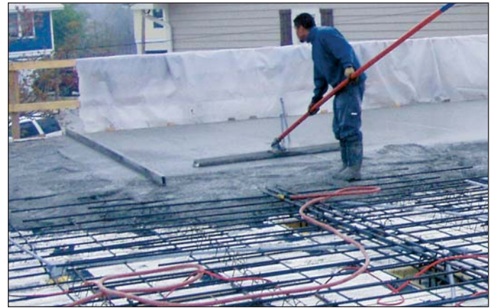
FIGURE 3. The elevated foundation employs a mix of commercial and residential methods. Grade beams are formed with wood, and reinforced with rebar as specified by the project engineer (top left). Vertical rebar is placed for connecting the grade beams to columns. After the beams are poured, reinforced columns are formed and poured using conventional basement wall forms. A rented commercial shoring system is set up to support the first-floor elevated slab (top right), and crews form the slab with plywood (bottom left). Then floor insulation, rebar, conduit, and blockouts for floor penetrations are placed, and the concrete is delivered (bottom right).
