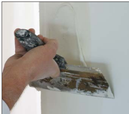
FIGURE 8. Red-iron beams (top) allow the creation of larger open spaces inside the houses. Wood-framed chases (above) can be used for architectural detail and to hide steel or ductwork. Plaster or drywall compound (left) applied directly to the concrete walls leaves the thermal mass of the concrete in contact with the occupied space.
