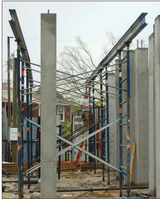
FIGURE 3. The elevated foundation employs a mix of commercial and residential methods. Grade beams are formed with wood, and reinforced with rebar as specified by the project engineer (top left). Vertical rebar is placed for connecting the grade beams to columns. After the beams are poured, reinforced columns are formed and poured using conventional basement wall forms. A rented commercial shoring system is set up to support the first-floor elevated slab (top right), and crews form the slab with plywood (bottom left). Then floor insulation, rebar, conduit, and blockouts for floor penetrations are placed, and the concrete is delivered (bottom right).
