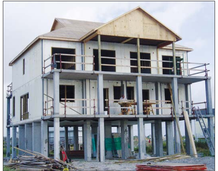
FIGURE 2. After the first elevated slab is set, crews can add as many as three more occupied stories in successive monolithic pours using the Wall Ties aluminum form system (left). Note the foam insulation (still exposed at this stage), which is placed against exterior forms before the pour and remains in place after forms are stripped. Pitched roofs are framed as a wood truss structure, on top of the main flat-topped concrete box (below).
